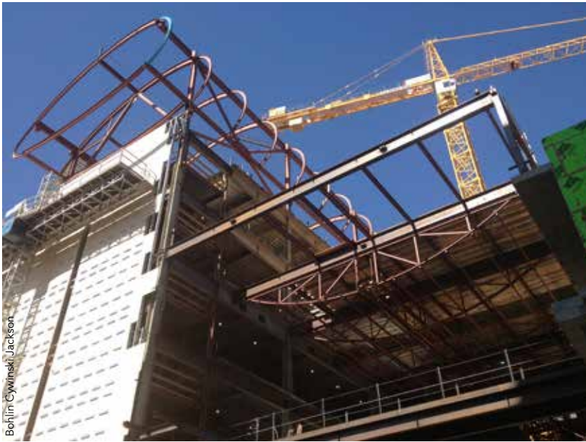
▲ The steel-framed mechanical penthouse uses roof beams whose radii vary from 109 ft, 8 in. all the way down to 3 ft, 4 in.
