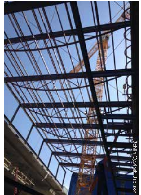
▲ The translucent glass ceiling is hung from steel trusses, which are in turn suspended from the roof girders.
