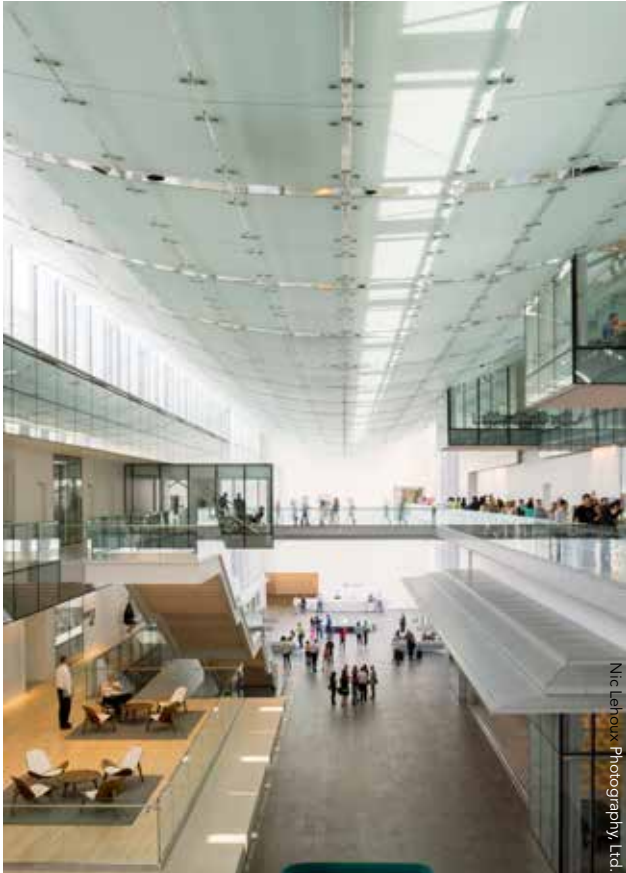
▲ ▼ Above the atrium, glass conference rooms cantilever into the space, and a gently curving ceiling of translucent glass is suspended below steel trusses supporting the skylight roof, mitigating the intense Utah sunlight and softening the interior space. There are three conference rooms—one at the third level that cantilevers 16 ft and two at the fourth level that cantilever 11 ft.
