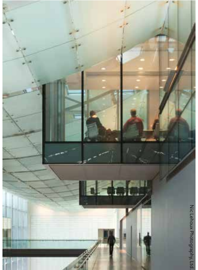
▲ ▼ Above the atrium, glass conference rooms cantilever into the space, and a gently curving ceiling of translucent glass is suspended below steel trusses supporting the skylight roof, mitigating the intense Utah sunlight and softening the interior space. There are three conference rooms—one at the third level that cantilevers 16 ft and two at the fourth level that cantilever 11 ft.
