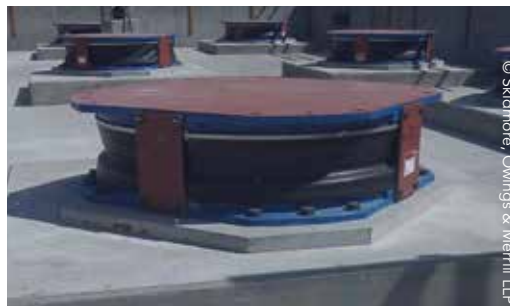
▲▲ The superstructure frame is supported on an energy-dissipating seismic isolation system above the lowest mat foundation. This system is made up of 69 triple concave-friction pendulum (TC-FP) bearings.
