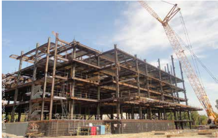
▲ The gravity steel-framed structure consists typically of a 3¼-in. lightweight concrete fill over 3-in. 20-gauge metal deck.
