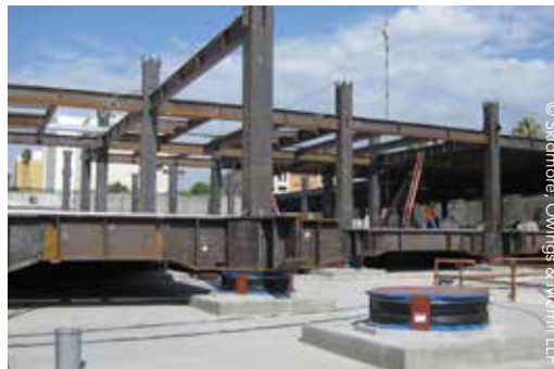
▲▲ The superstructure frame is supported on an energy-dissipating seismic isolation system above the lowest mat foundation. This system is made up of 69 triple concave-friction pendulum (TC-FP) bearings.
