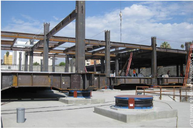
▲ The superstructure frame is supported on an energy-dissipating seismic isolation system above the lowest mat foundation level. This system is made up of 69 triple concave-friction pendulum (TC-FP) bearings.
