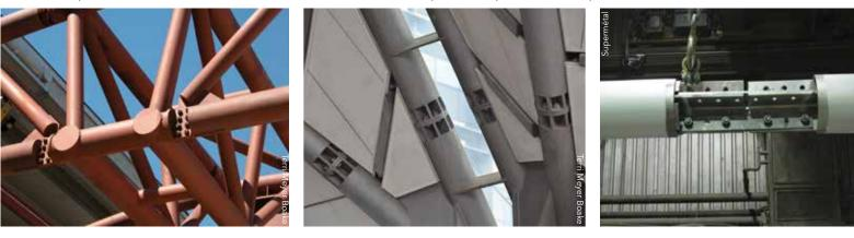
**16.** For reduced visibility of large splices, consider hidden or discreet connections. If the intention is to simply make the splices appear less visible, given either the level of exposure of the AESS or budgetary restrictions, there are two other very effective cost-saving options:
