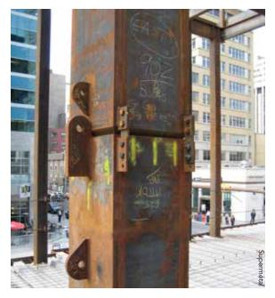
Tip 6 – Weld complex nodes in the shop and bolt on-site as much as possible. The joint shown in contact bearing was machine finished. All field joints were bolted. All shop welds were CJP.
