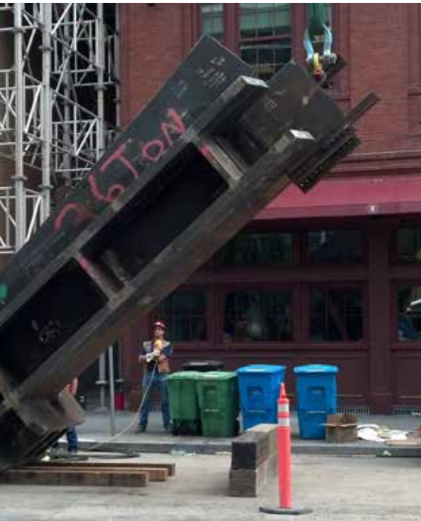
▲ The building uses approximately 9,000 tons of structural steel.
