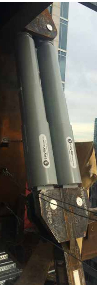
◀ ▲ The external damped megabrace system eliminated the need for the TMD and introduced an uplift mechanism at the base of the megacolumns to eliminate tension demands in the foundation. Instead of stiffening the building, the design actually reduces stiffness, elongating the building period to reduce seismic demands accordingly.
