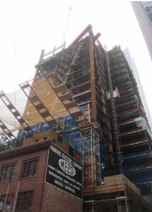
▲ A cantilevered safety net protects an adjacent building.
