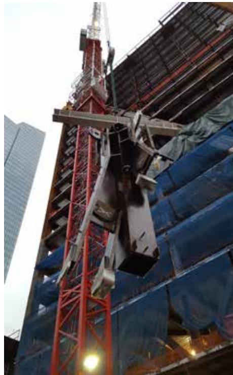
▲ Steel could only be erected from Fremont Street, and an assist crane was used for heavier picks at the back of the building.
