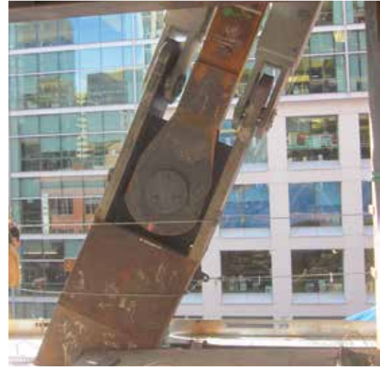
▲ ▼ Each of the externally exposed megabraces in the office levels is 200 ft to 250 ft long, extending across multiple floors to the meganodes. The megabraces comprise three braces in parallel: a primary brace with a secondary brace on either side.
