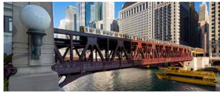
**THE WELLS STREET BRIDGE** is the longest double-deck, double-leaf, bascule bridge built over the Chicago River, and only one of two remaining bascule bridges in the city of Chicago that carries both automobile and transit (Chicago Transit Authority elevated trains) on two levels.
