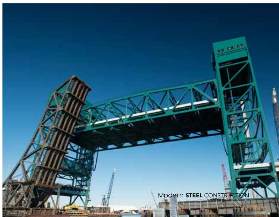
Because rock was too deep to rest the drilled shaft foundations on, the foundations were predicted to experience some settlement with time. Settlement can be an issue for any bridge, but is of particular concern for movable bridges because of the precise tolerances required to ensure operation without binding. Jacking brackets were designed into the towers to allow them to be jacked under full, dead load to compensate for the settlement.
