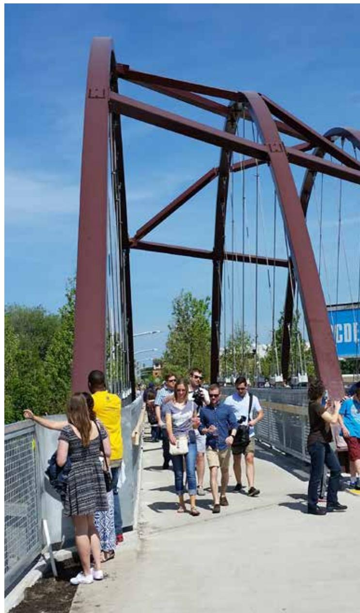
structure, including modal and dynamic analysis. The existing girders were spliced together at the piers for continuity and retrofit steel was added to the existing plate girders where needed due to the deterioration that had taken place over the past 100 years. Lateral earth loads were reduced by the use of geo-foam, allowing the existing abutments to be completely reused.
