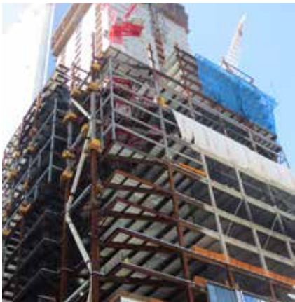
The steel-framed WTC 3, under construction.
