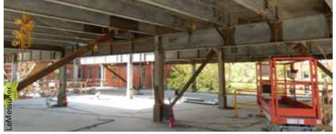
▲ The design team elected to consider the existing moment frame structure as a reserve system, which was analyzed independently according to an array of damage scenarios.
