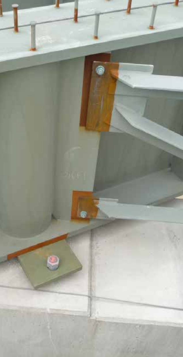
▲ An SPBS used for a cross frame connection along a highly skewed bent line.
