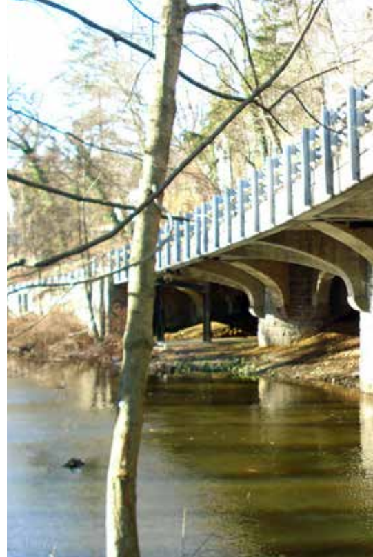
◀ The bridge's concrete-encased brackets and core.
