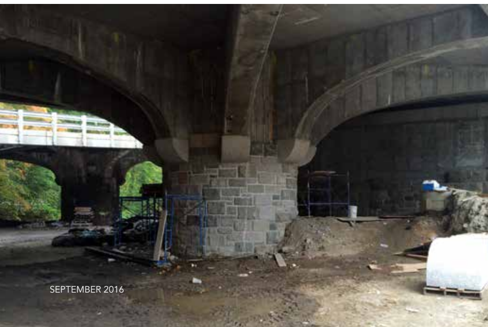
◀ Existing bridge in the background; replicated structure in the foreground.
