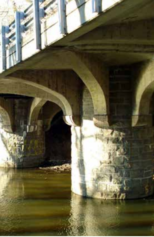
▲ The bridge's uniquely shaped piers gave it its Mushroom Bridge nickname.
