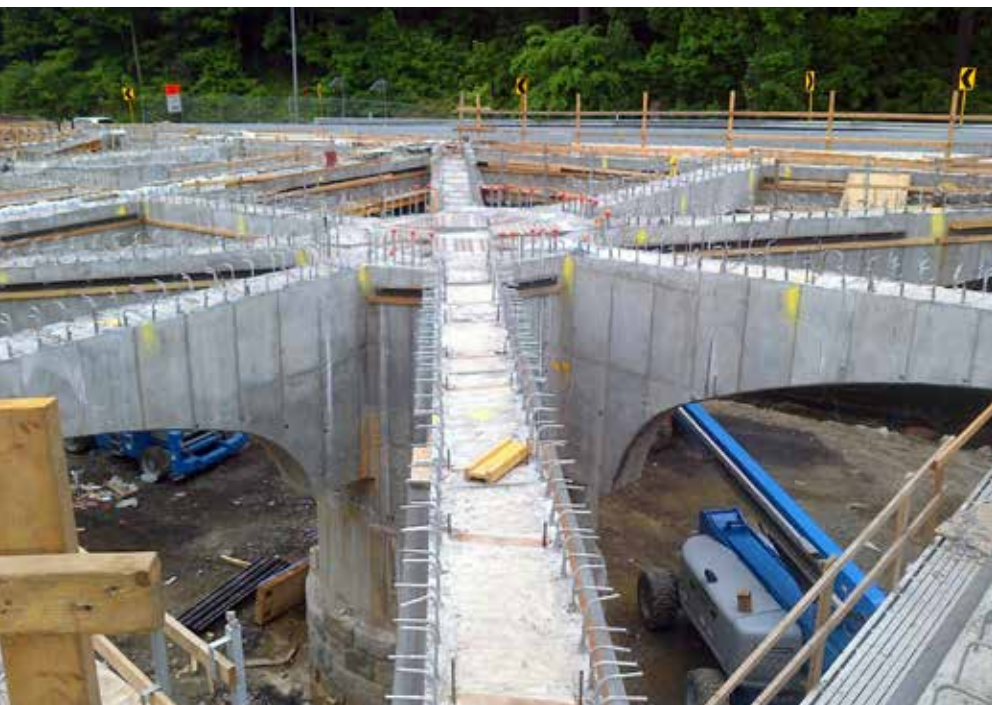
▲ The partially erected Mushroom Bridge, showing steel core and steel brackets.
