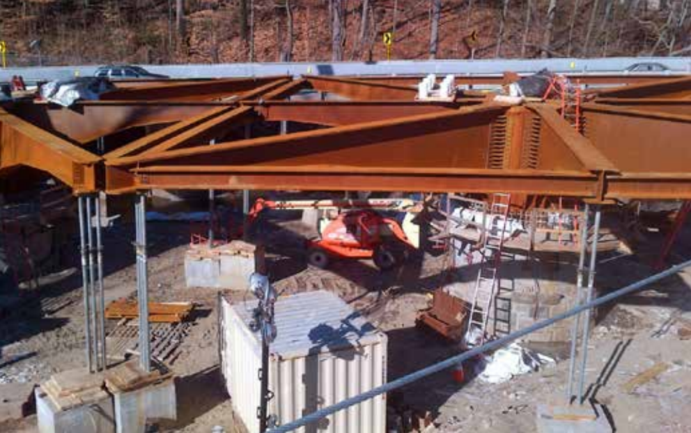
▲ The partially erected Mushroom Bridge, showing steel core and steel brackets.
