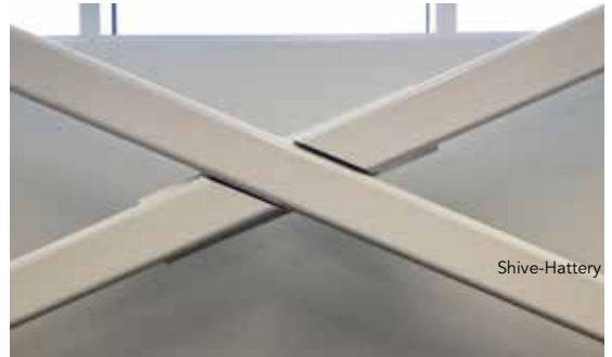
▲ The X-bracing was typically HSS5×5×3/8.
