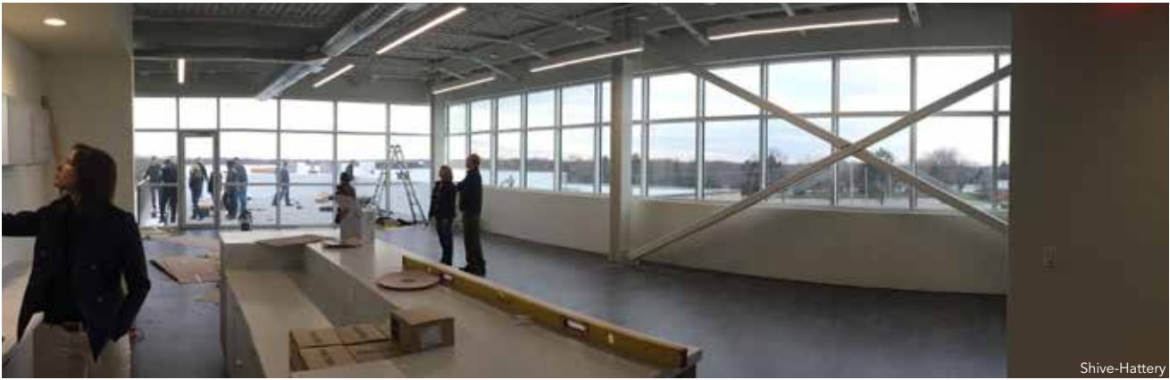
▲ The X-bracing in the breakroom during construction.
