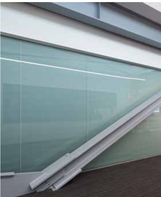
▼ Structural braced frames are expressed sculpturally.
