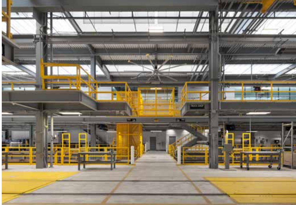
▲ Large skylights fill the maintenance area with diffused natural daylight.
