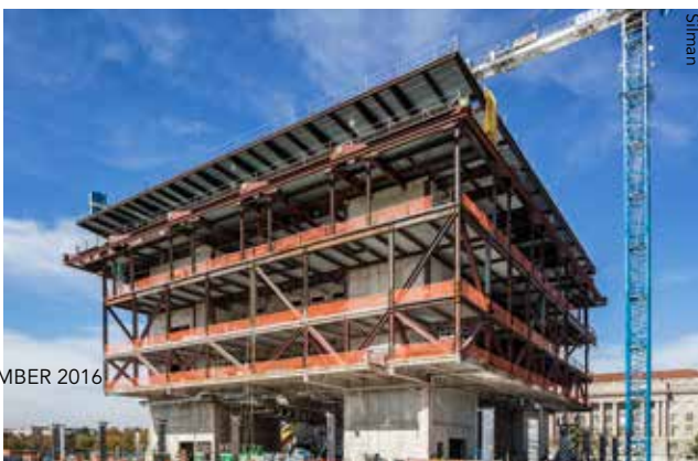
▼ The project uses just over 4,000 tons of steel in all.
