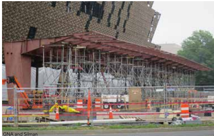
▲ The porch canopy structure, under construction.
