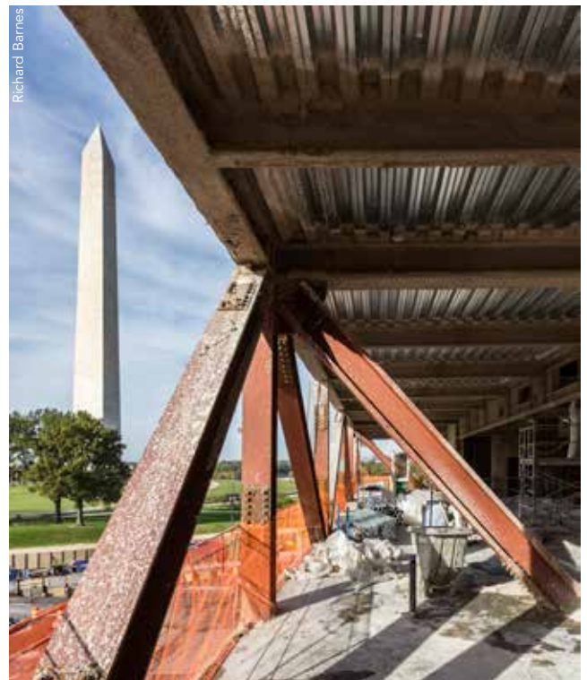
▼ The level 2 platform with perimeter vertical steel trusses.
