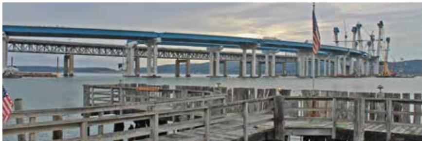
▲ One of this year's many SteelDay events was a presentation on the new Tappan Zee Bridge north of New York City. Members of the design team provided insight on the project to a crowd of nearly 80 at a venue overlooking the bridge itself.
