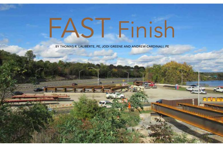
▲ At the lay-down area, temporary or "mock" abutments were constructed to match existing bridge substructures, which were reused for the proposed bridge. **WITHIN 15 MONTHS** from the notice to proceed for design, four bridge superstructures carrying Route 8 over Lindley Street and Capitol Avenue in Bridgeport, Conn., were fully replaced and open to the public.
