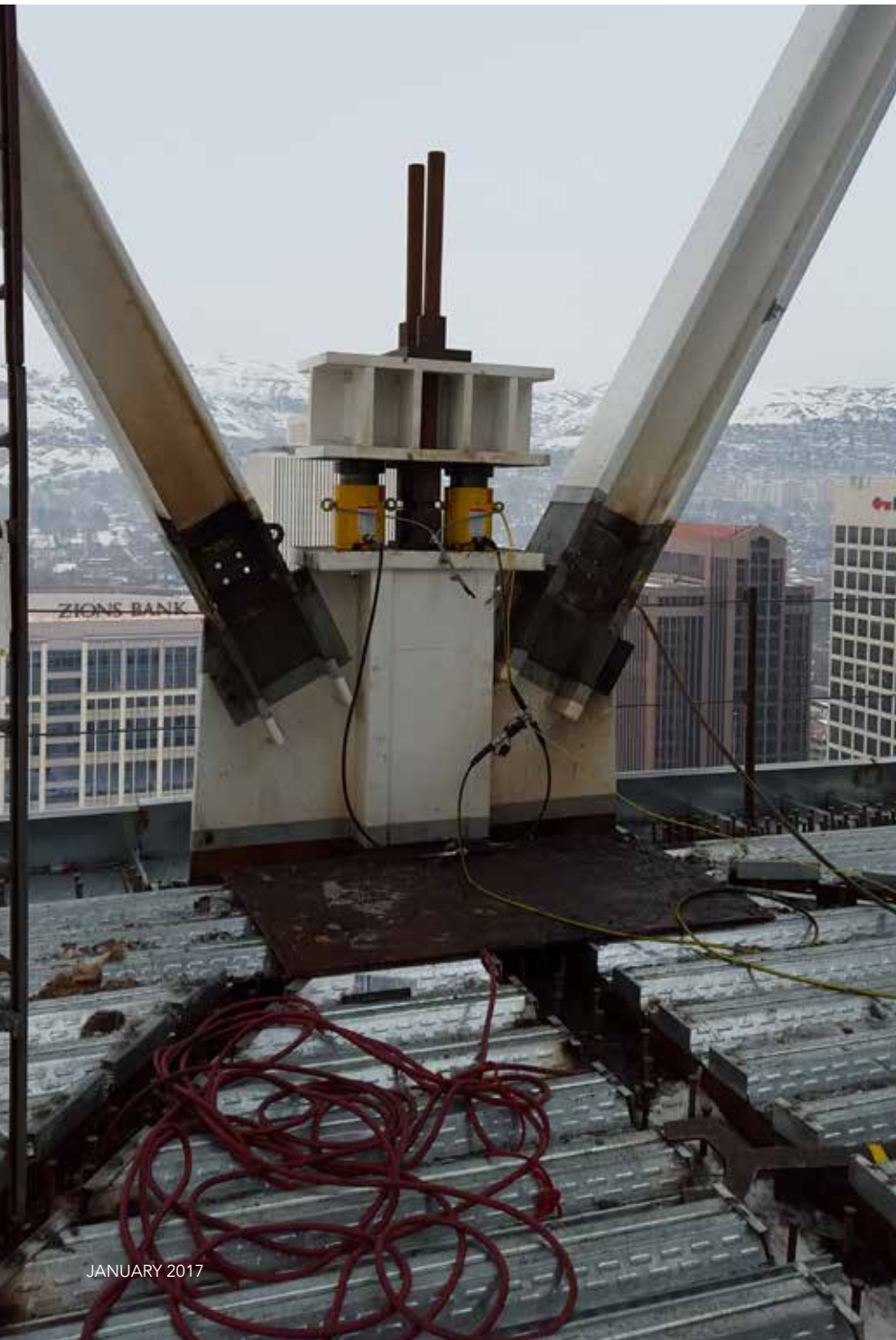
◀ Jacking adjustments at the roof node.
