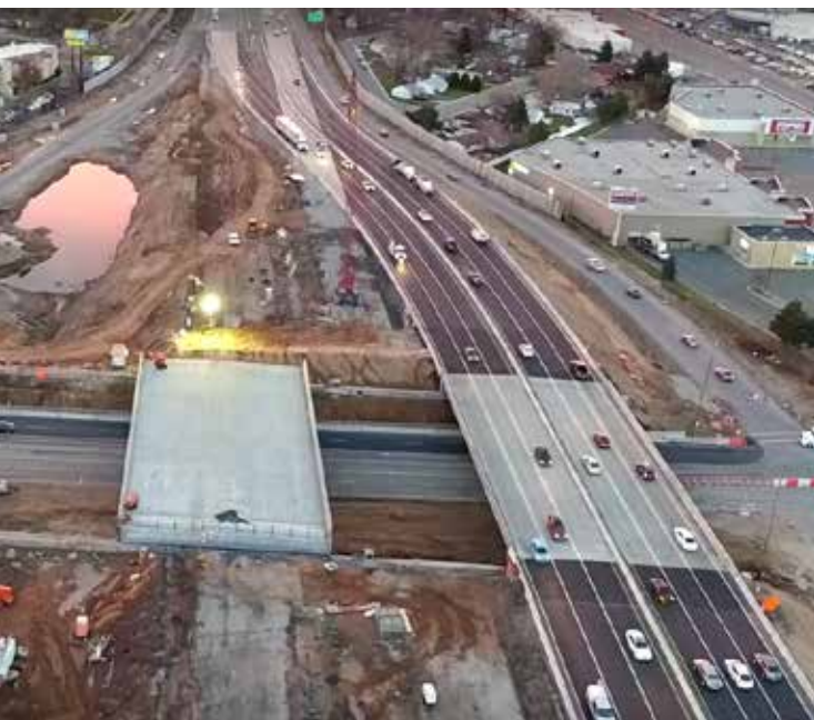
▼ The southbound bridge was used as a shoofly while the northbound bridge was slid into its final position.
