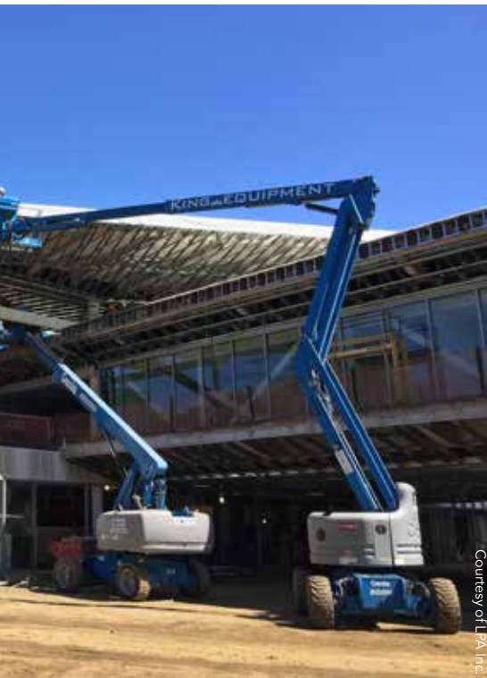
▲ The butterfly-form roof under construction. Rainwater is collected through the cantilevered scupper into the sustainable garden below.
