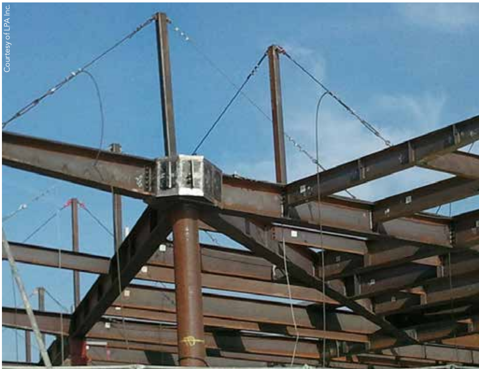
▲▼ Steel box plate connector hubs connect as many as six cantilevered beams across a single column.
