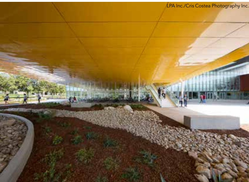
▼ The column-free area beneath the skybox.
