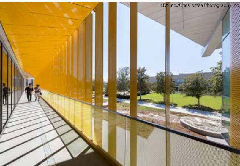
▲ An exterior walkway is shaded by perforated metal panels.
