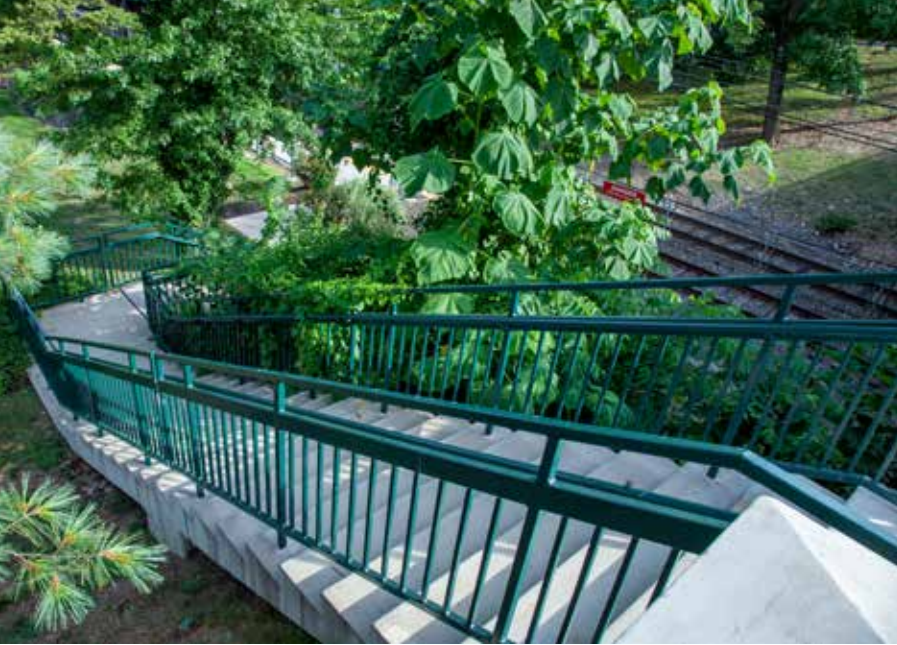
◀ Stairs from street level down to the SEPTA tracks.
