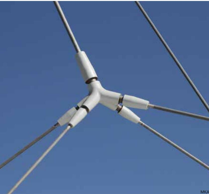
▲ A closeup of a single turnbuckle casting on the San Ysidro Land Port of Entry project.
