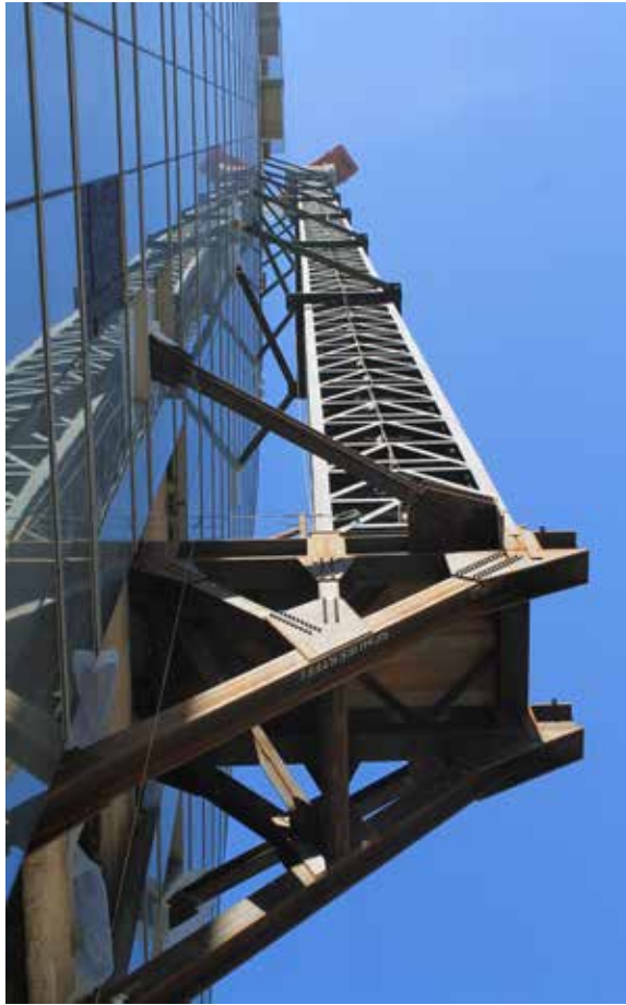
▲ A temporary cantilevered steel structure supported the tower crane on the building's north side, so the crane wouldn't be required to land on the sidewalk/street.
