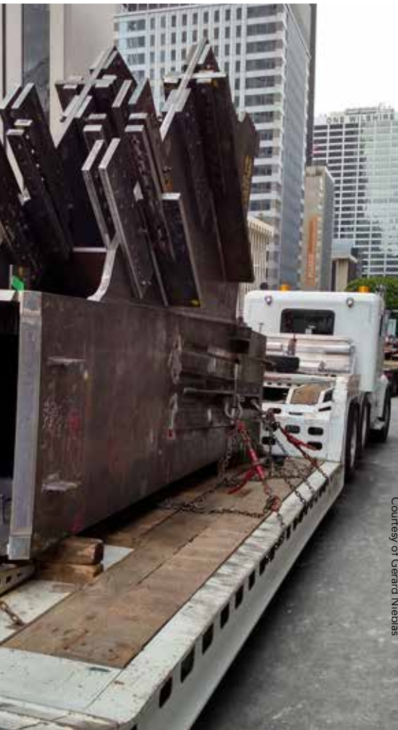
▲ A temporary cantilevered steel structure supported the tower crane on the building's north side, so the crane wouldn't be required to land on the sidewalk/street.
