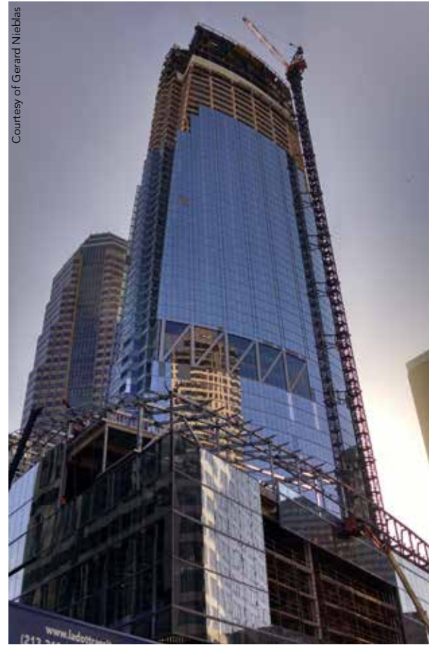
▲ A temporary cantilevered steel structure supported the tower crane on the building's north side, so the crane wouldn't be required to land on the sidewalk/street.
