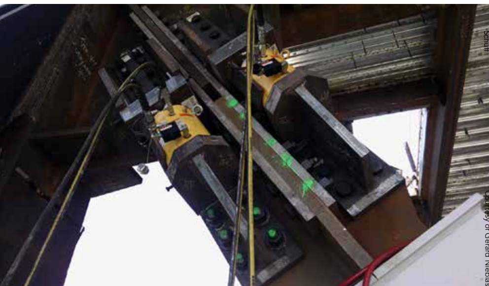
▲ The team jacked each of the upper BRBs with a pre-compression force of 1,000 kips.
