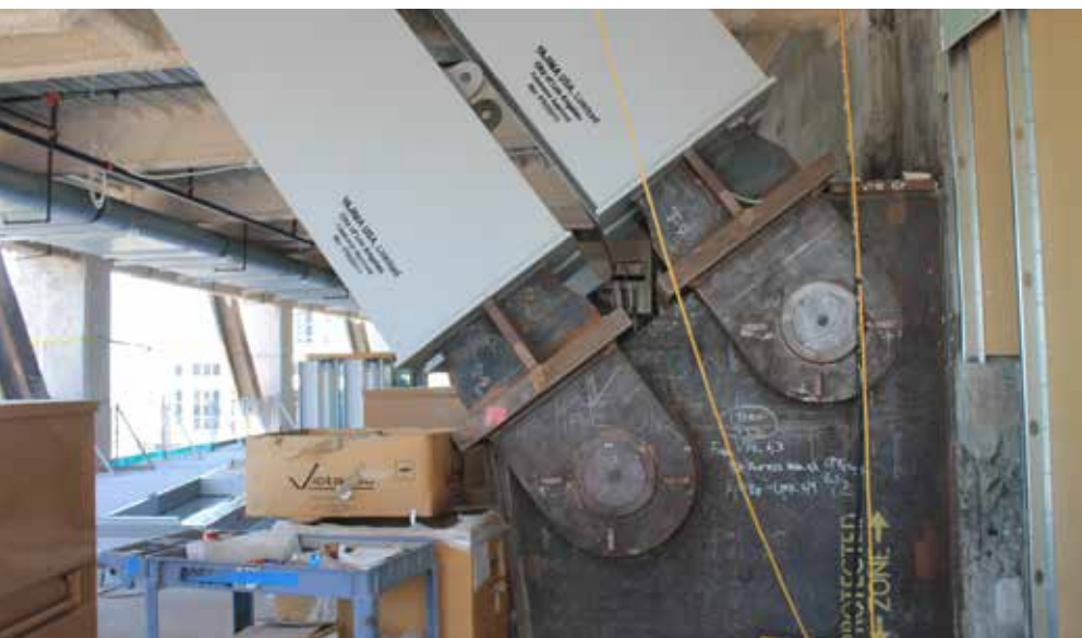
▲ The team jacked each of the upper BRBs with a pre-compression force of 1,000 kips.
