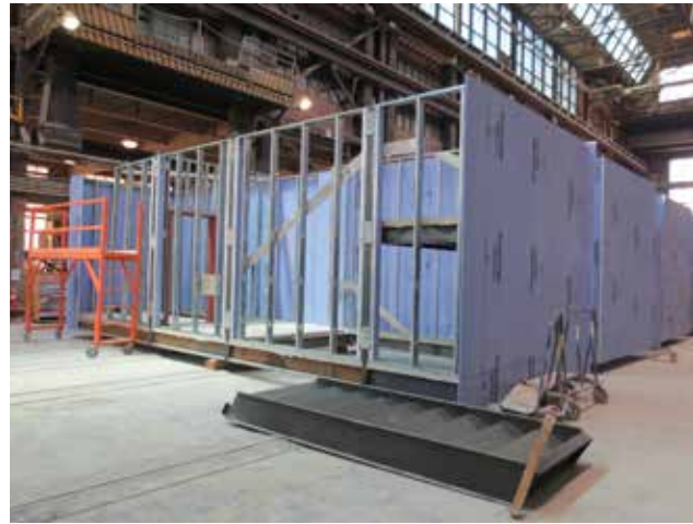
▲ A volumetric module coming together, incorporating framing, fixtures and cladding.
