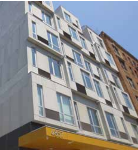
▲ The Stack, a modular residential project in New York.
