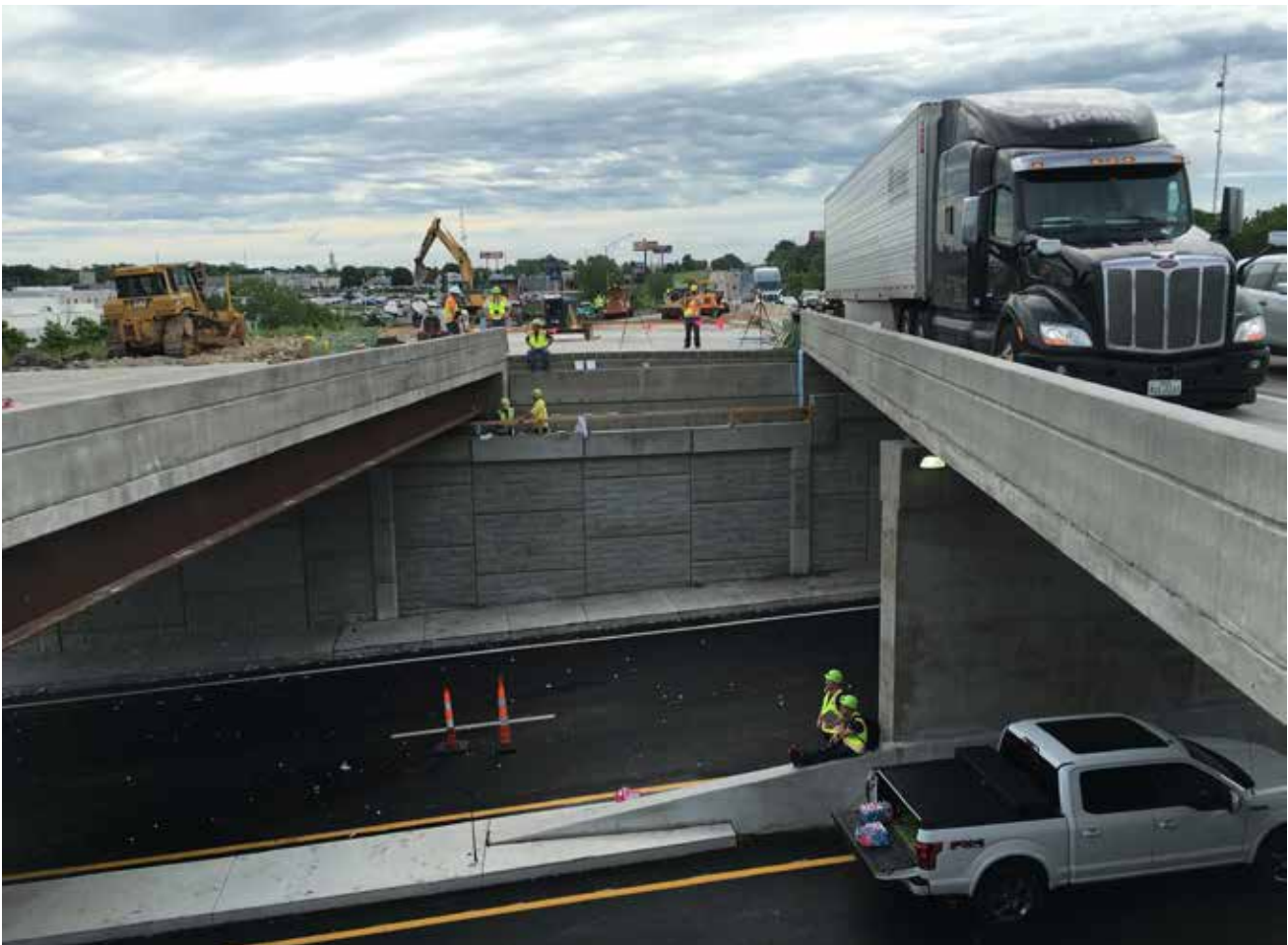
▲ The 355-ton westbound I-70 Bridge over Garth Ave. was slid 36 ft. ▼ Slide in progress for the westbound I-70 bridge over Rangeline.
