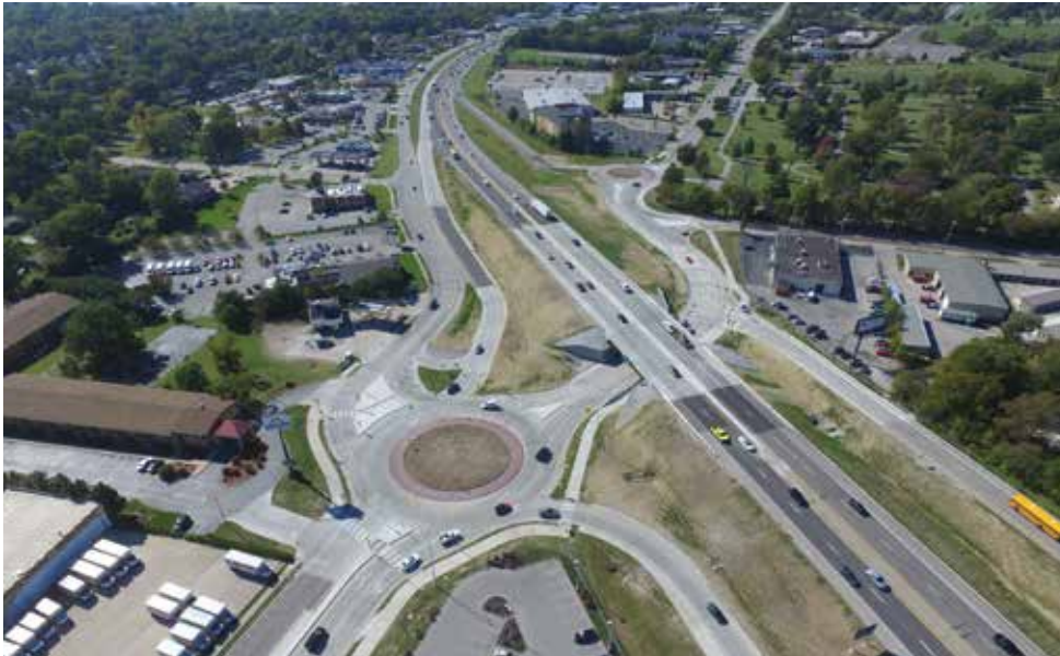
◀ An aerial view of the I-70 bridge over Business Loop, which replaced two existing bridges.
