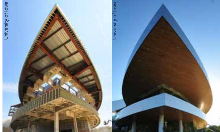
▲ Before and after cladding shots of the underside of both cantilevers.
