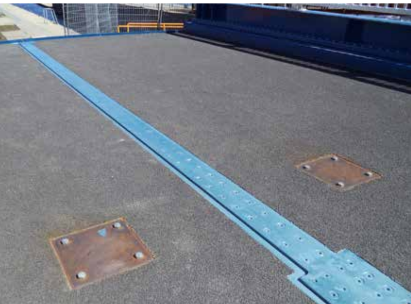
▲ A view of the longitudinal bolted splice between the orthotropic steel deck panels before asphalt was added. The panels were delivered with an anti-skid waterproofing membrane that was preinstalled by the fabricator for durability and worker safety during the wet winter months.
