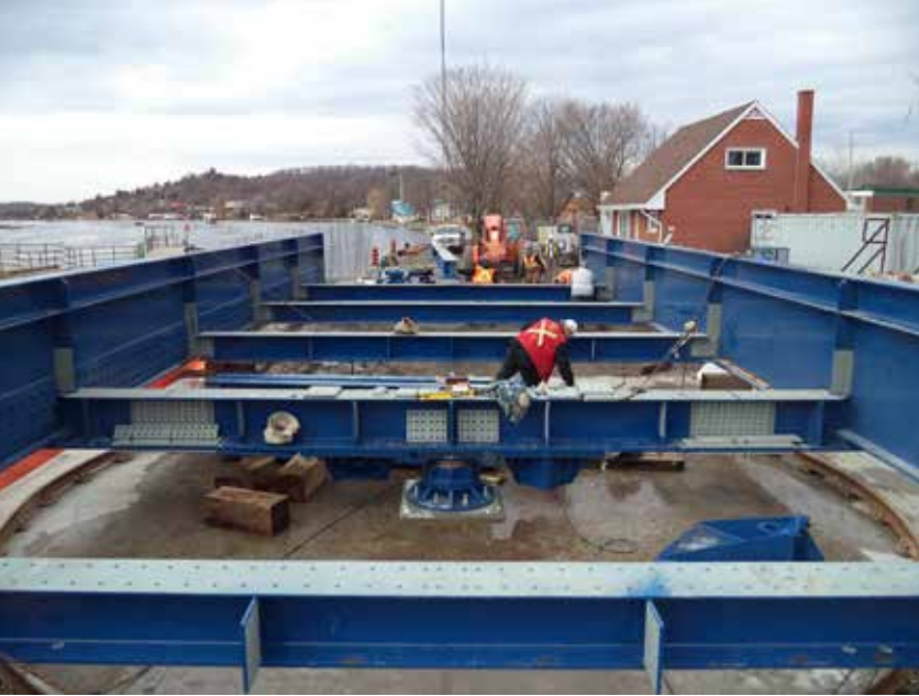
◀ A view of the steel superstructure prior to installing the OSD. The transverse floor beams of the OSD were used as a template to drill matching holes in the superstructure above.
