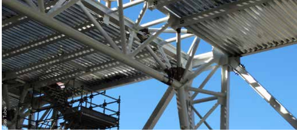
▲ ▲ The tri-chord trusses, under construction. Translucent panels above the trusses allow sunlight to penetrate the building.
