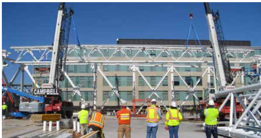
▲ Lifting the first truss into place. ▼ The fabricator built the trusses as if they were for a bridge, not a building.
