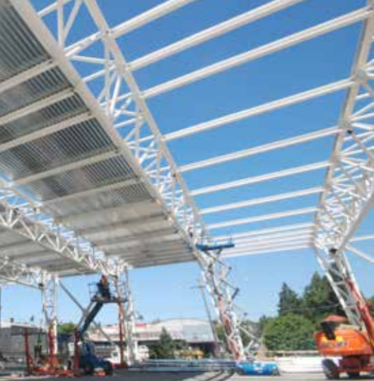
▲ ▲ The tri-chord trusses, under construction. Translucent panels above the trusses allow sunlight to penetrate the building.
