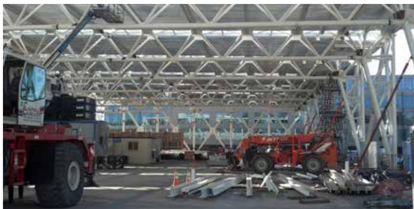
▲ Lifting the first truss into place. ▼ The fabricator built the trusses as if they were for a bridge, not a building.
