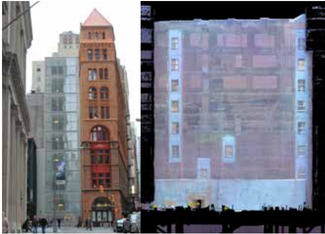
▲ Laser scanning was used for New York's Fulton Center, which incorporated the historical landmark Corbin Building. (The project was featured in last month's IDEAS 2 Awards coverage.)
