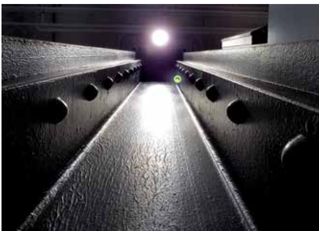
▲ Many historic structures originally used rivets for resisting connection loads.
