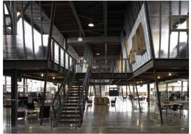
▲ A structural renovation project in Des Moines, the new headquarters for Two Rivers Marketing Group, incorporated a new steel-framed mezzanine within the existing walls of a former GM warehouse. (See "Second Chance" in the February 2007 issue.)
