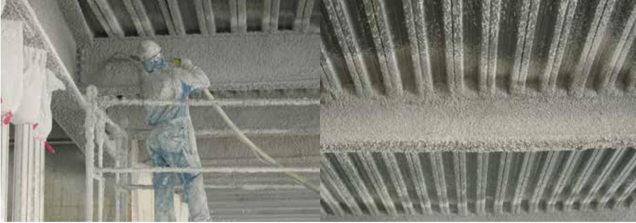
▲ The two-hour assembly ratings in UL Design D982 can be used with any UL-certified spray-applied fire-resistive material (SFRM) with thickness “sufficient to provide a one-hour Unrestrained Beam Rating.”
