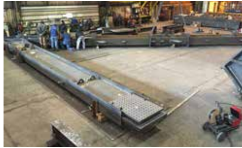
◀ A type 1 truss plate girder and node, connected in the shop.
