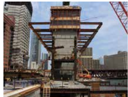
▶ At the lower levels where the forces are significant, the goal was to minimize the number of erectable pieces in order to reduce construction cost and optimize the schedule. The lower levels (below the full-floor office levels) incorporate 54 major pieces weighing between 26.5 tons and 31 tons and up to 68 ft long. The main laydown area was located to the west of the building on the overbuild atop existing rail lines, as well as to the south in areas that would become public spaces.
