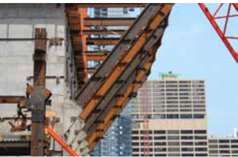
▲ The 60-ft diagonal sections of the type 1 trusses projecting from the core.
