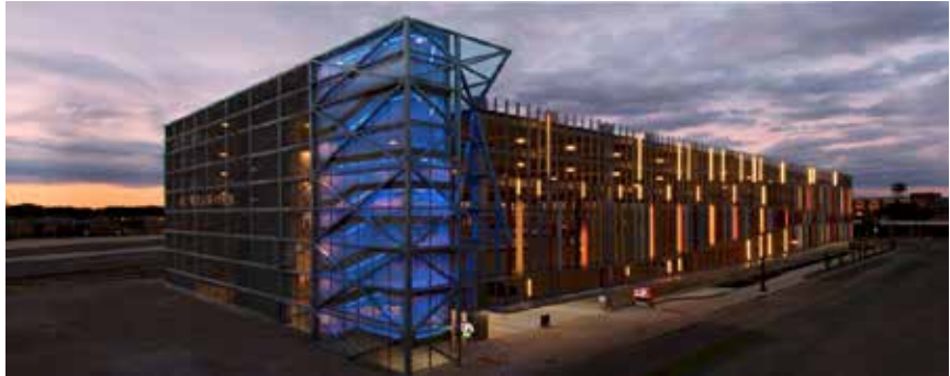
▲ The new Goodale Parking Garage in Columbus, Ohio, was the Transportation winner in AGA's 2017 Excellence in Hot-Dip Galvanizing Awards. The project used 275 tons of structural steel, fabricated by Wanner MetalWorx (an AISC member and certified fabricator).
