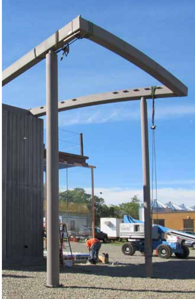
▲ A full-size mockup including the precast cladding, glazing and canopy was built.
