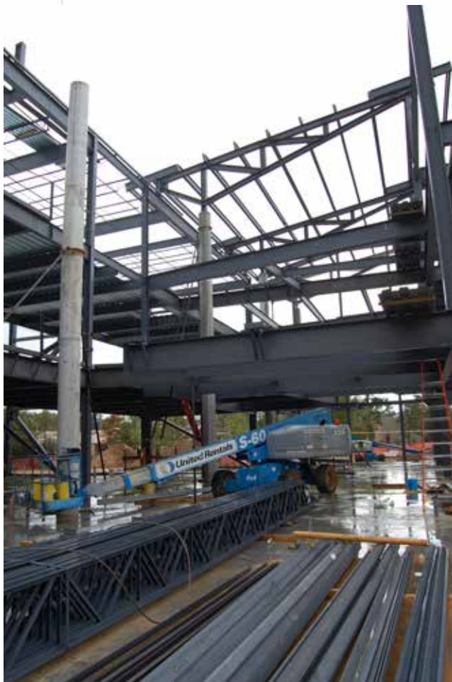
▶ The complicated geometry of the building, both in the 2D floor plans and in the multiple roof elevations and slopes, made this project an ideal candidate for using structural steel and a BIM workflow.
