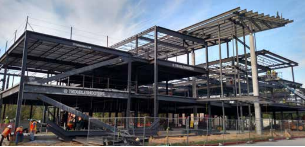
▲ Each roof truss balances on a 40-ft-tall exposed, unbraced concrete column.
