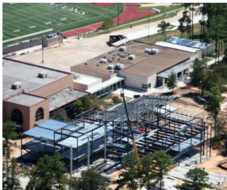
▶ The complicated geometry of the building, both in the 2D floor plans and in the multiple roof elevations and slopes, made this project an ideal candidate for using structural steel and a BIM workflow.
