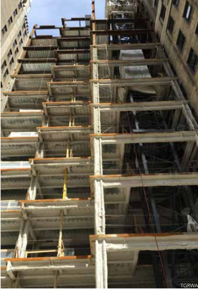
▲ Framing view from the back side of the building.
