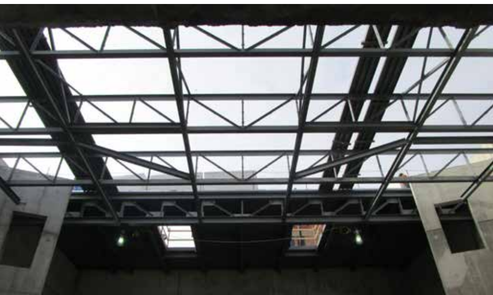
▲ ▼ Erecting the theater roof framing. Wide-flange steel trusses span 70 ft across the width of the theater, and lighter trusses comprised of WT chords and double-angle web members span over the house.
