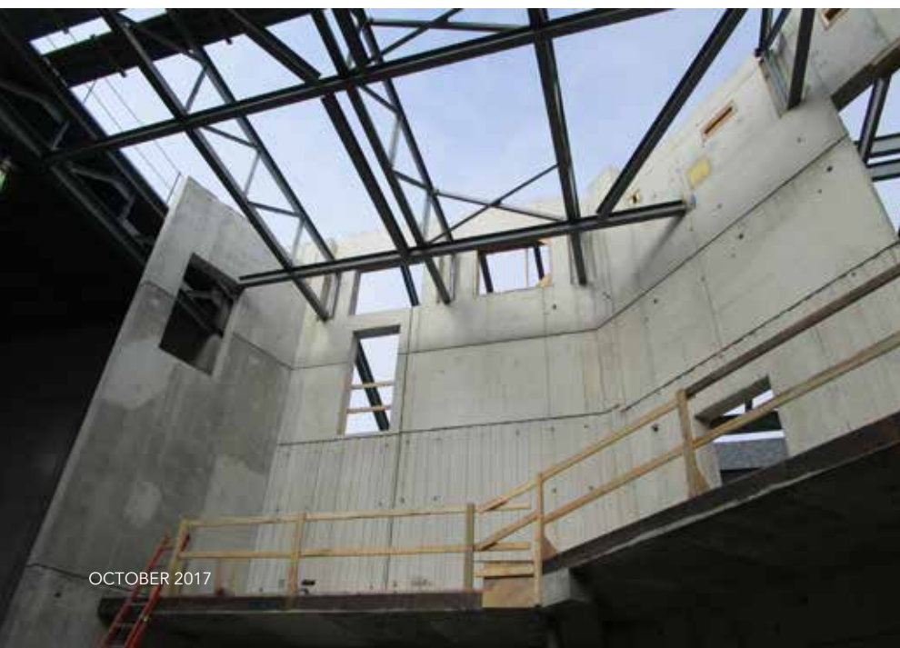
▲ ▼ Erecting the theater roof framing. Wide-flange steel trusses span 70 ft across the width of the theater, and lighter trusses comprised of WT chords and double-angle web members span over the house.
