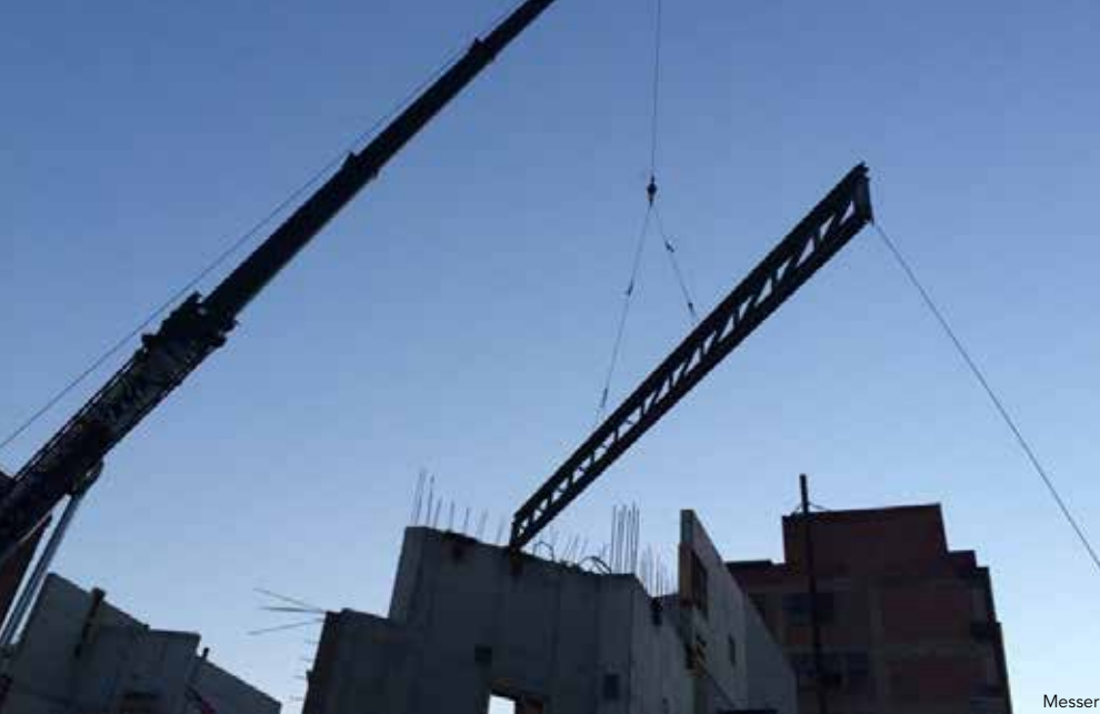
◀ Erecting the proscenium truss.
