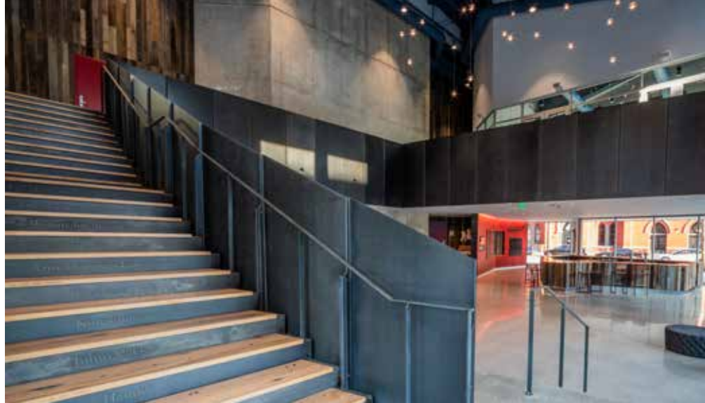
▲ ▼ Steel plate railings in the lobby. The steel stair risers feature laser-cut play titles from the Shakespearean cannon.
