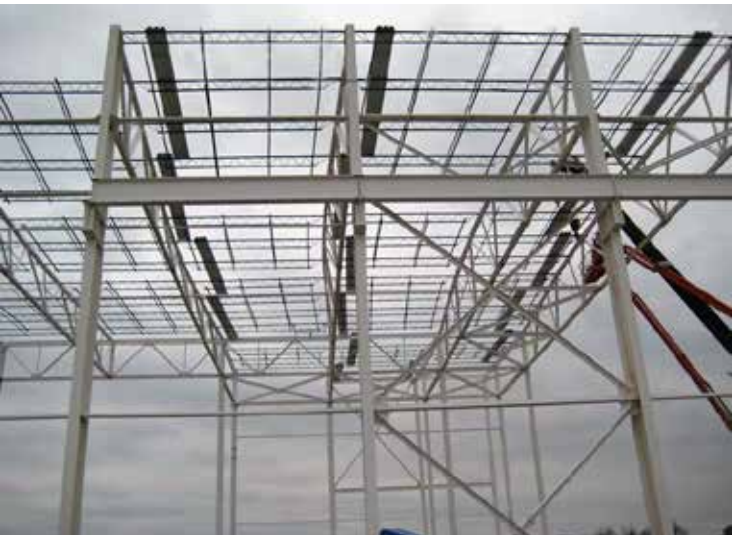
▲ Figure 4. The erector was totally unaware of the structure's stability requirements until the roof structure shifted, as shown here.
