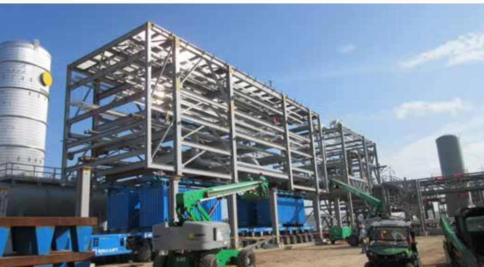
▲ Transporting a module via SPMT. ▼ Setting a process module in place.
