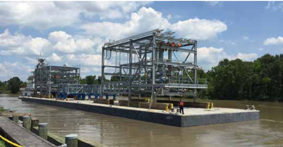
◀ Barging in a process facility module.
