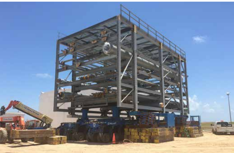
▲ Transporting a module via SPMT. ▼ Setting a process module in place.
