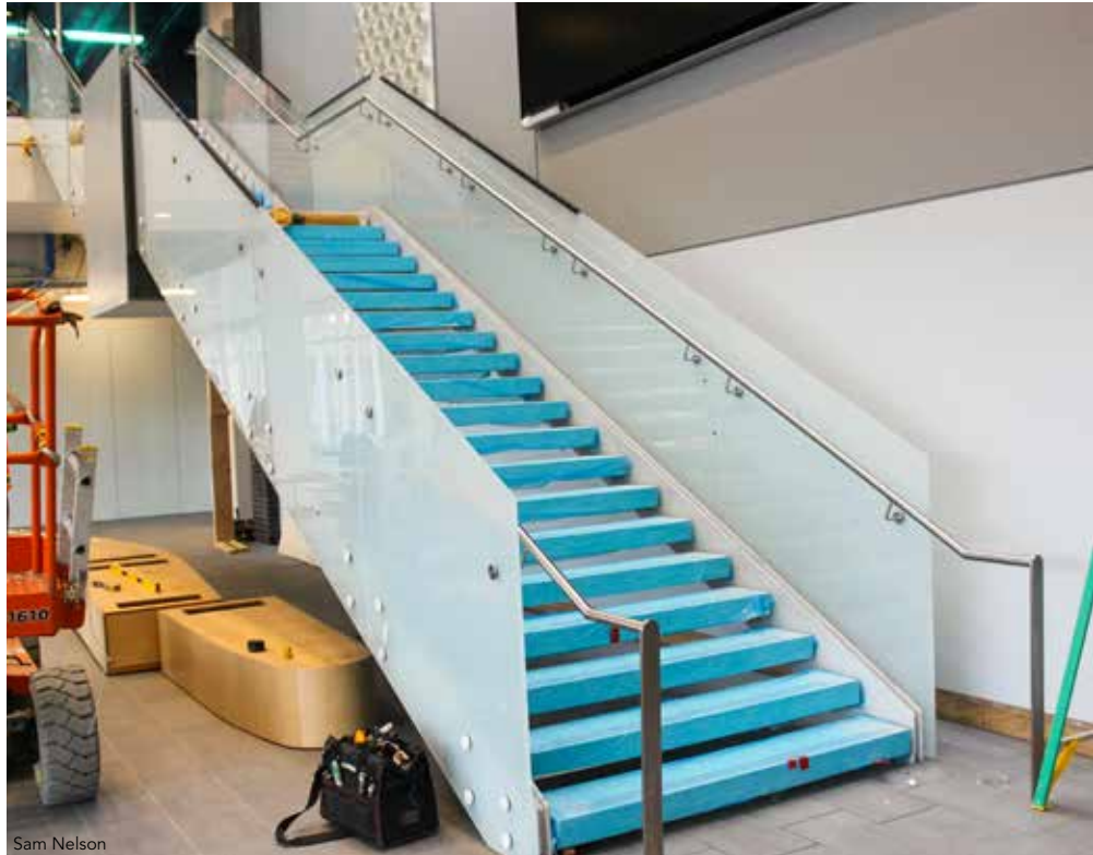
▲ The feature stair connecting levels 1 and 2.
