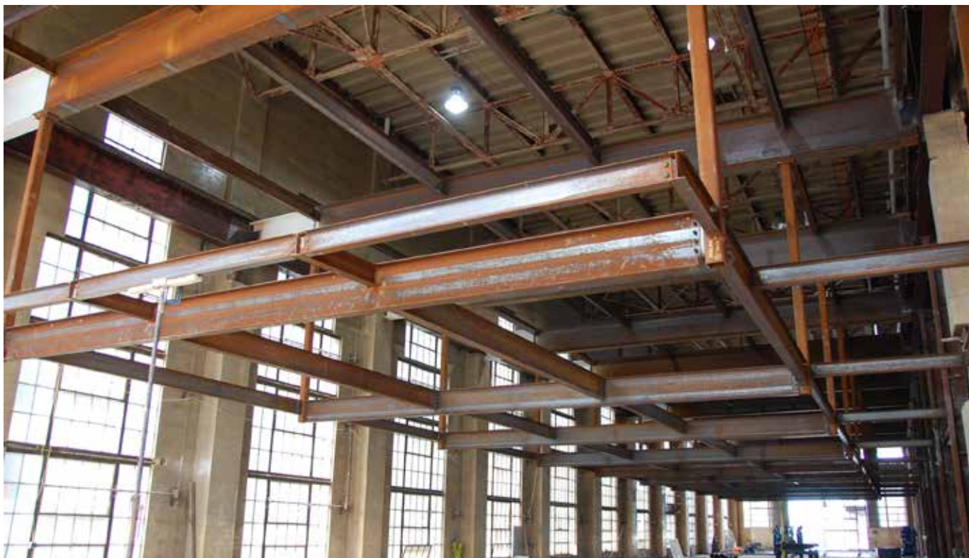
above: New fourth-floor steel was attached to the crane rail in the building's turbine hall, with third-floor steel hung from the bottom.
