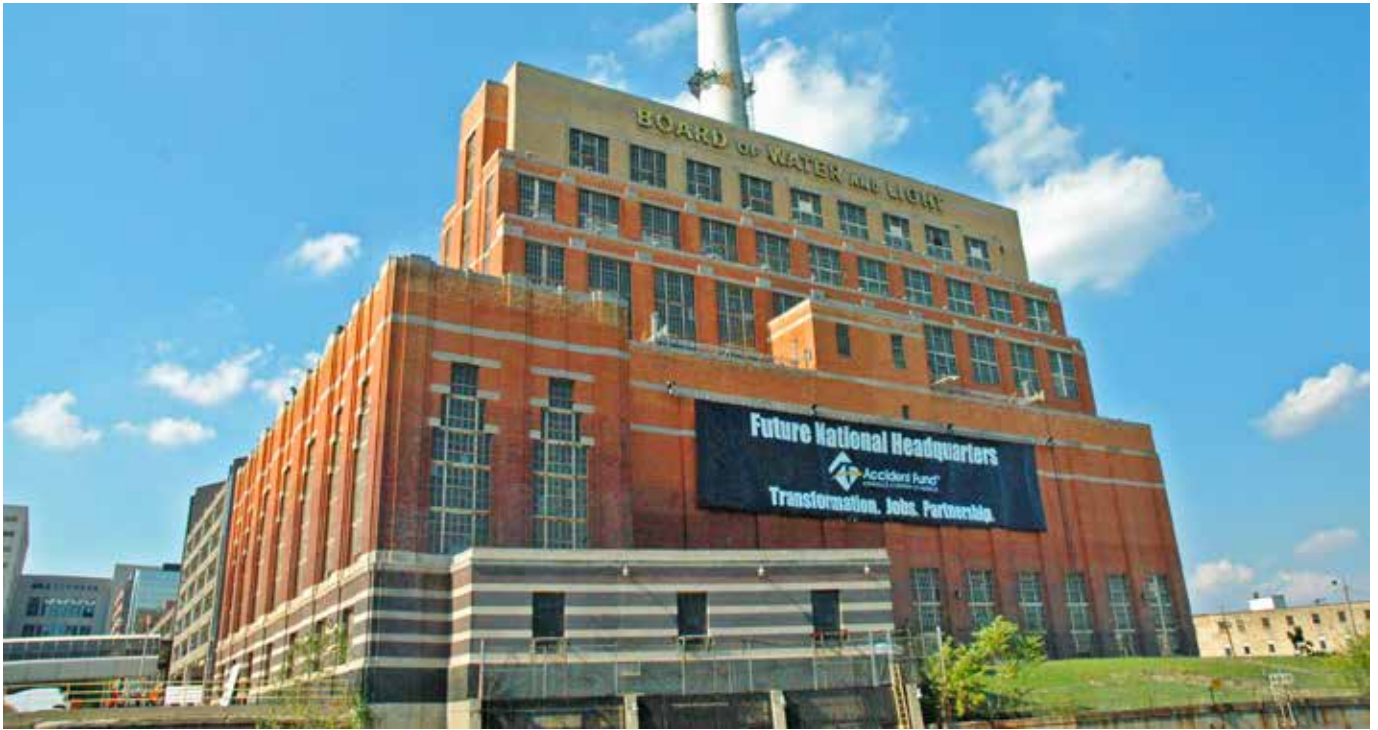
below: Lansing, Michigan's 1939 Ottawa Street Power Station encompassed a major structural renovation. This model shows new steel members in red and existing members being incorporated into the new structure in gray.
