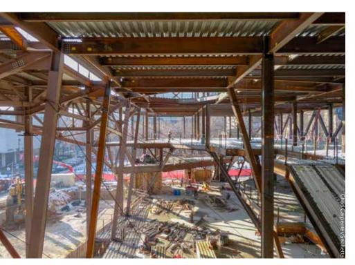
above: Construction of the atrium, with "spanning wall" members visible in the distance.
