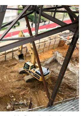
below: Truss erection at the southwest entrance. The corner column at the far right is a temporary support.
