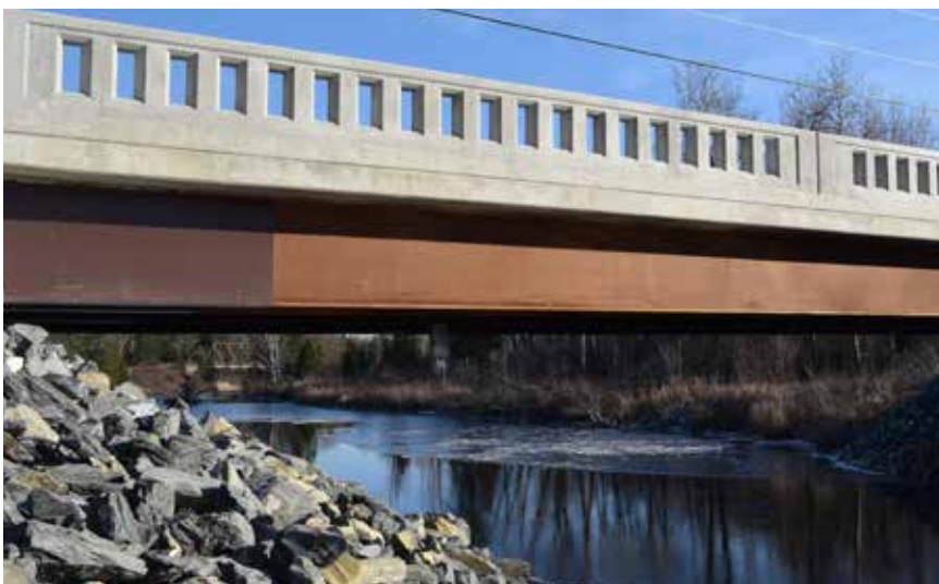
Bridge #5160, which carries Main St. over the Little Madawaska River in Stockholm, Maine, was repainted with a PAS system.
