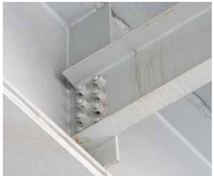
A Connecticut DOT project—I-75 over Starr Ave. in Danbury—was repainted in 2002 with a PAS system. After 15 years in service, minimal rust has been experienced.
