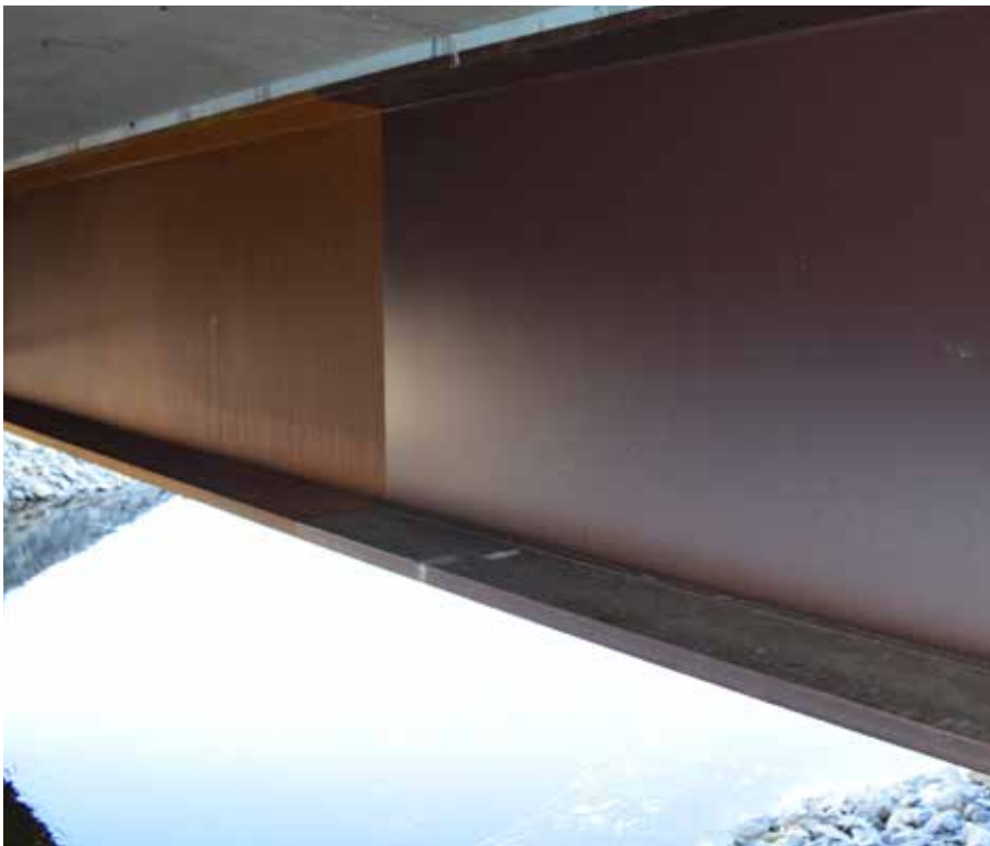
The Maine bridge project is a simple-span design with four steel girders spanning about 100 ft.
