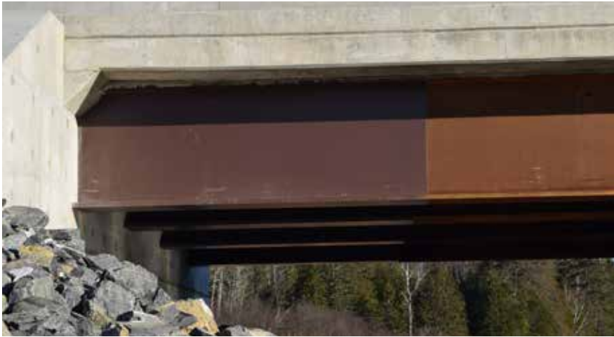
A close-up view of one of the painted beam ends on the Main St. bridge project.
