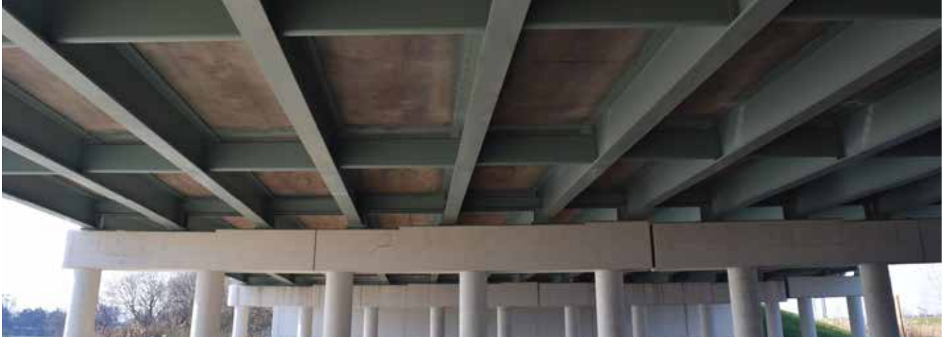
A Michigan DOT project—West Road over I-75 in Woodhaven, Mich.—was repainted with a PAS system in 2017.
