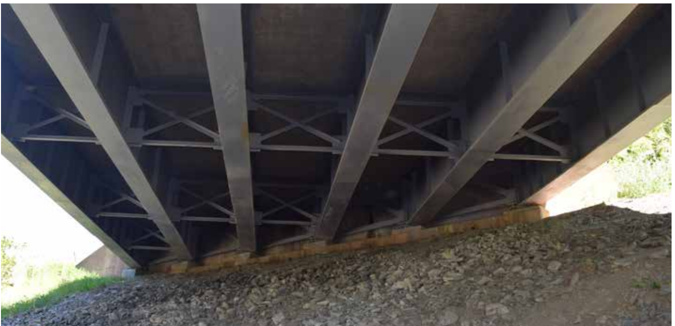
A Virginia DOT project—I-64 over Simpson Creek in Clifton Forge—was repainted with a PAS system in 2005 and has experienced minimal rusting after 12 years in service (above photos and bottom-left photo on opposite page).
