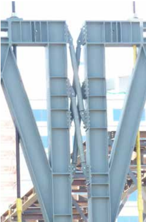
A rocking frame system with energy-dissipating couplers between the frames.
