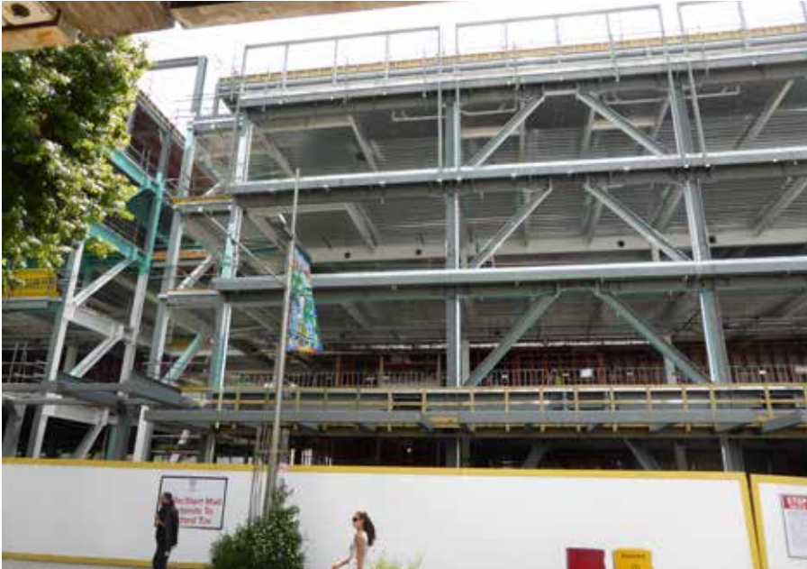
An EBF with replaceable links (left) and a close-up of a link in an inverted-V braced frame (right).
