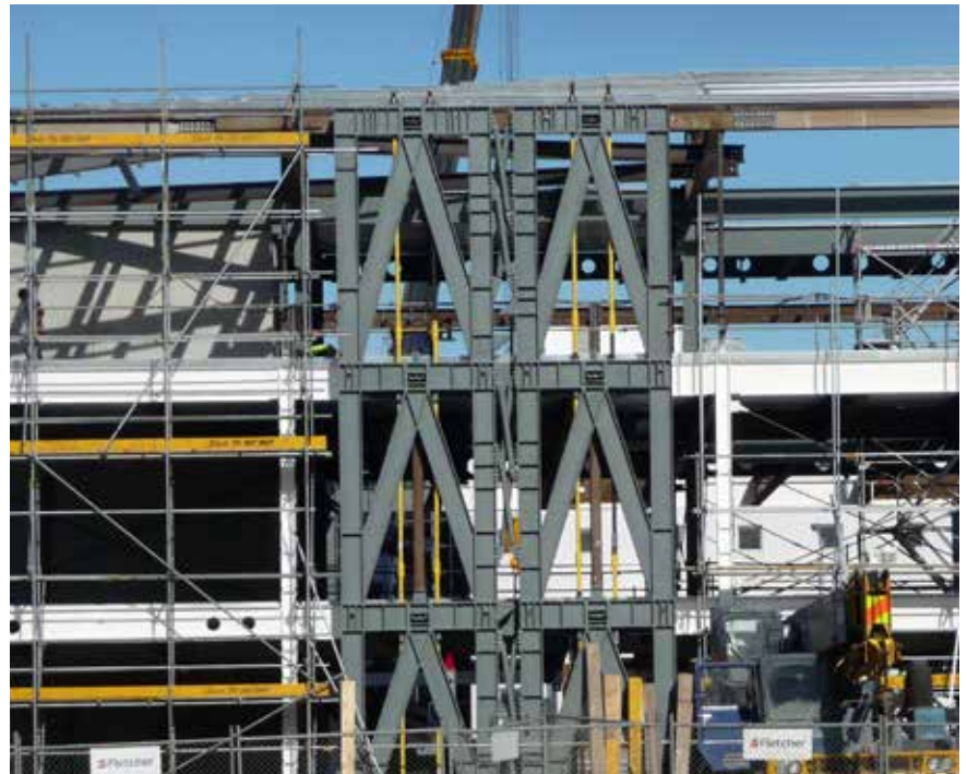
A rocking frame system with energy-dissipating couplers between the frames.
