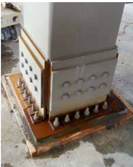
A base friction connection (left) and a completed bidirectional moment friction connection (right).
