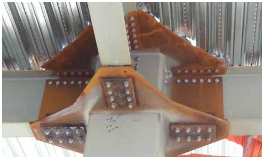
A base friction connection (left) and a completed bidirectional moment friction connection (right).
