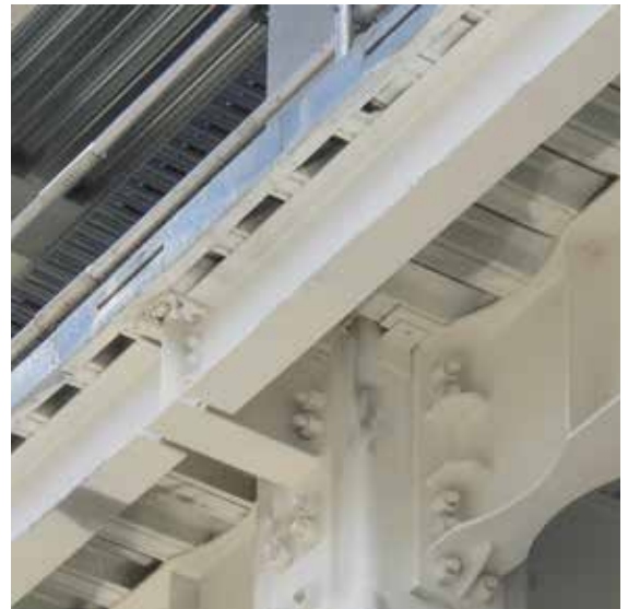
A space moment frame (left) and a close-up of an RBS connection in the form of a bolted end-plate to moment-resisting connection to a square steel section (right).
