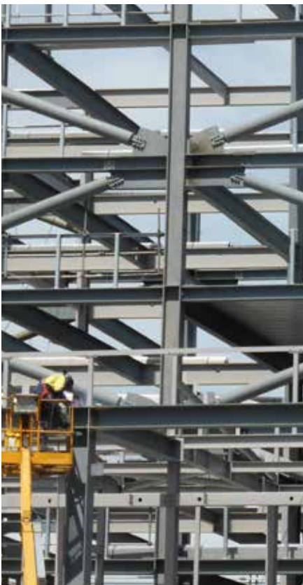
A BRB frame (left) and a column connection at mid-bay of the frame (right).
