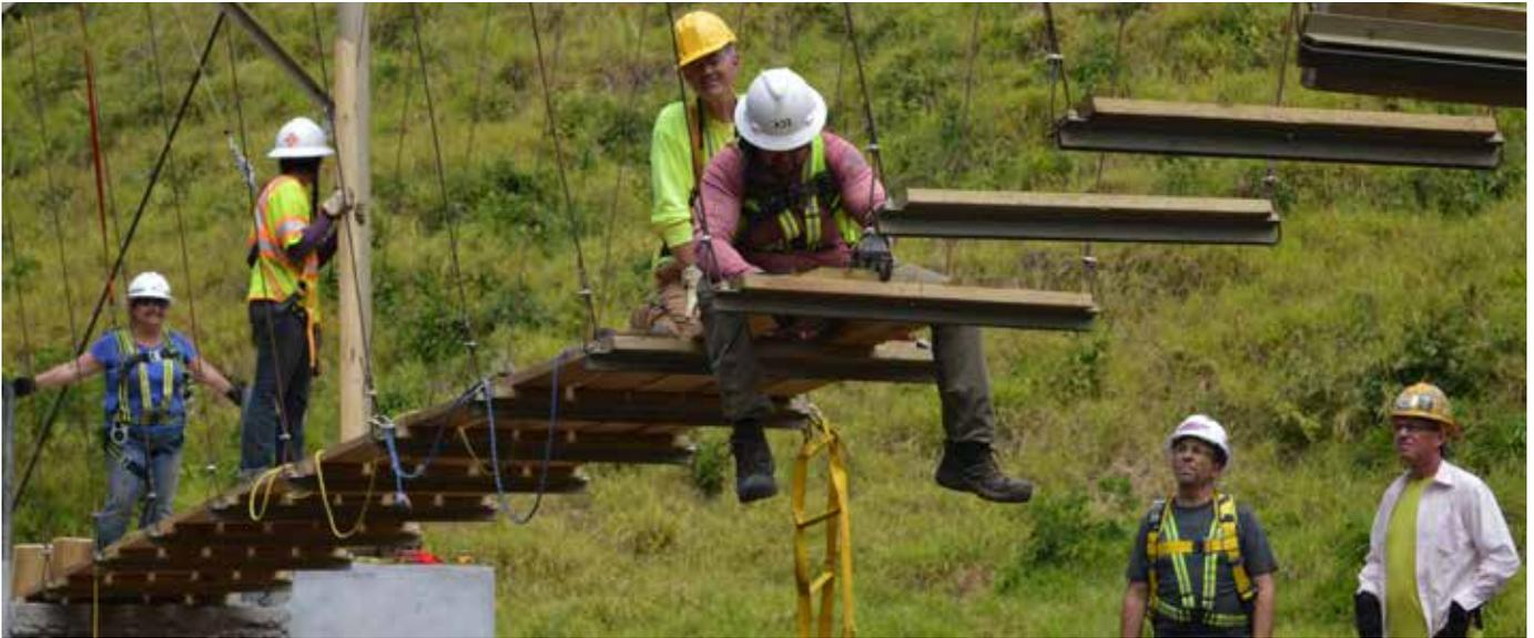
Carter Bearden and Gary Kinchen installing decking near the middle of the bridge span.
