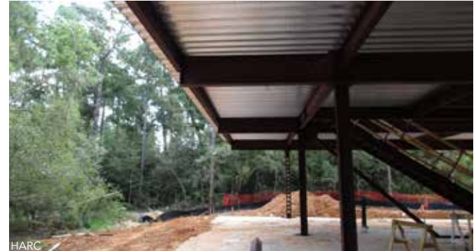
Wide-flange girders span the 62-ft direction of the building, and 24-ft composite steel beams span between the girders.
