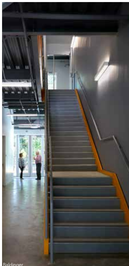
The steel-framed stairs, installed.
