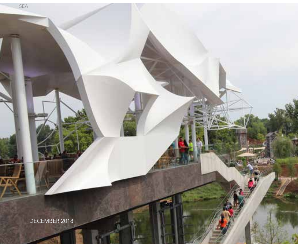
The centerpiece of the boathouse is a fiberglass canopy supported by HSS, that serves as the roof for the upper-most pavilion level.
