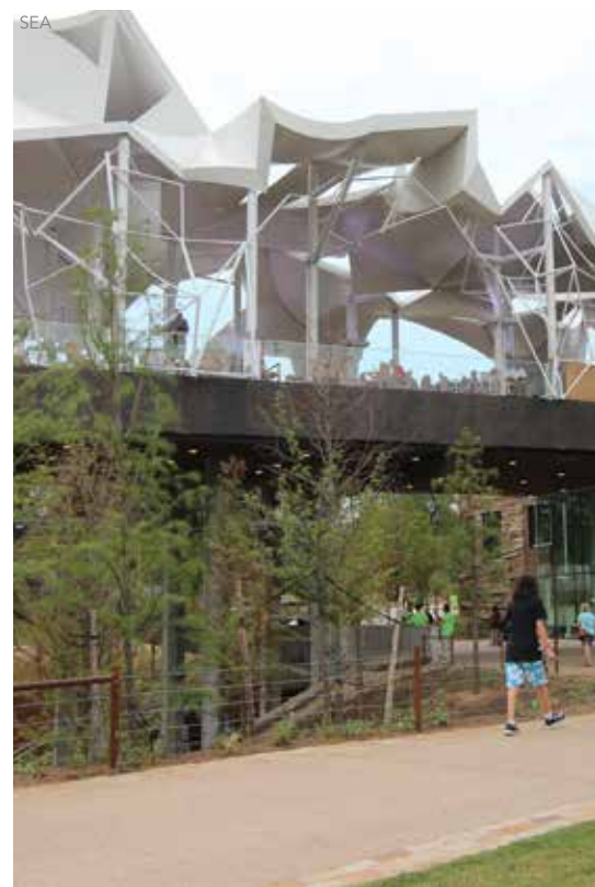
The centerpiece of the boathouse is a fiberglass canopy supported by HSS, that serves as the roof for the upper-most pavilion level.
