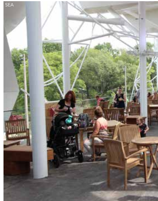
The centerpiece of the boathouse is a fiberglass canopy supported by HSS, that serves as the roof for the upper-most pavilion level.
