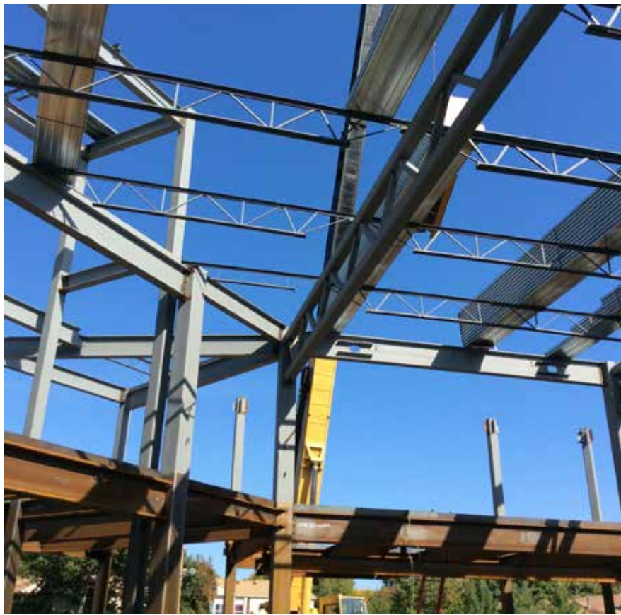
above: With a total area of 84,000 sq. ft and a height of 44.5 ft, the main structure employs an ordinary moment-resisting frame system.
