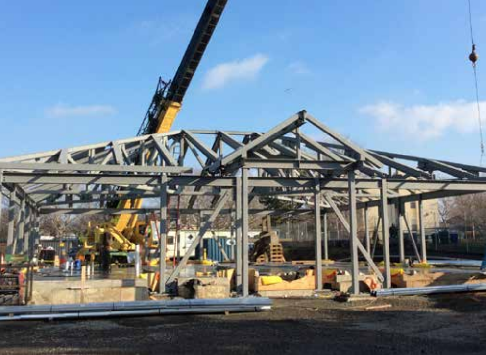
above: The administrative building uses roughly 50 tons of steel.
