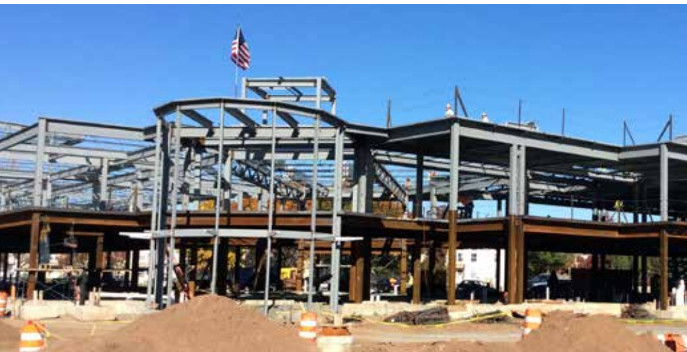
above and below: The main school building uses roughly 600 tons of structural steel framing.
