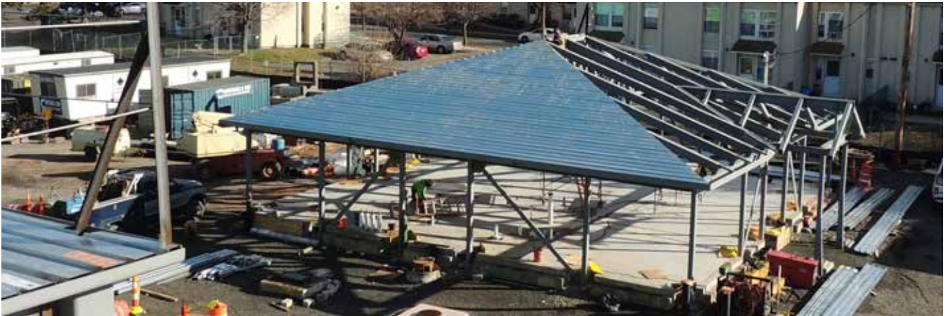
below: The framing for the smaller, administrative building consists of a combination of HSS sections and wide-flange beams, with the main lateral force-resisting system made of bracing built up in the perimeter walls.
