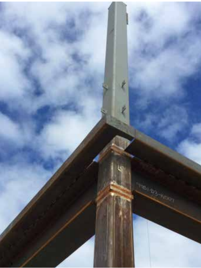
above: With a total area of 84,000 sq. ft and a height of 44.5 ft, the main structure employs an ordinary moment-resisting frame system.
