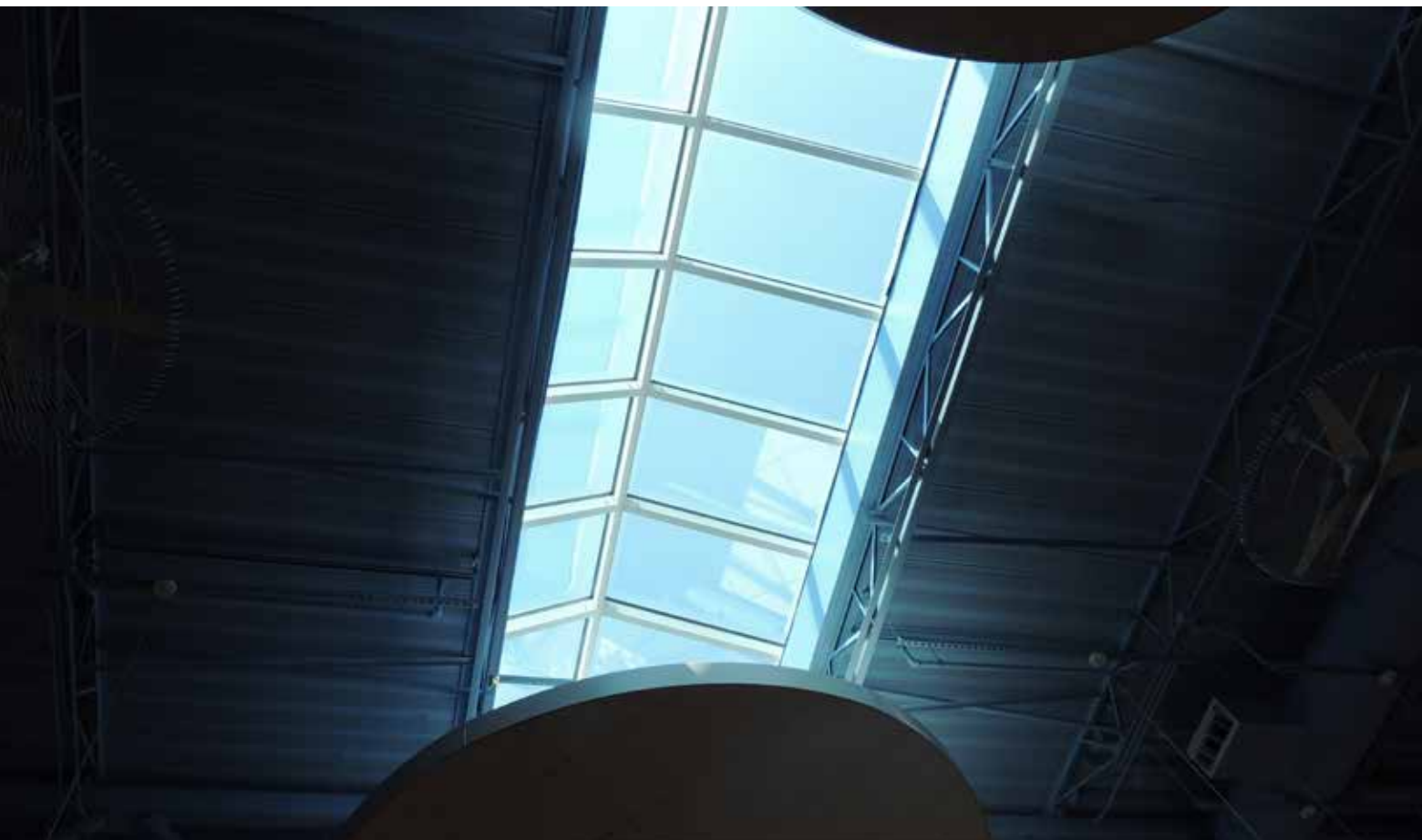
below: Joist framing at the skylight.
