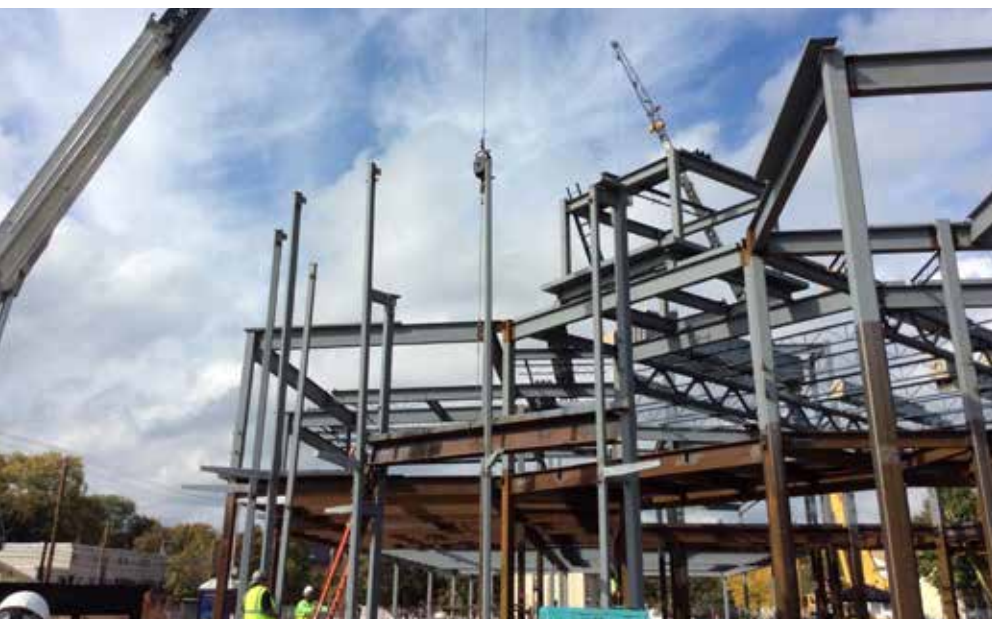
above and below: The main school building uses roughly 600 tons of structural steel framing.
