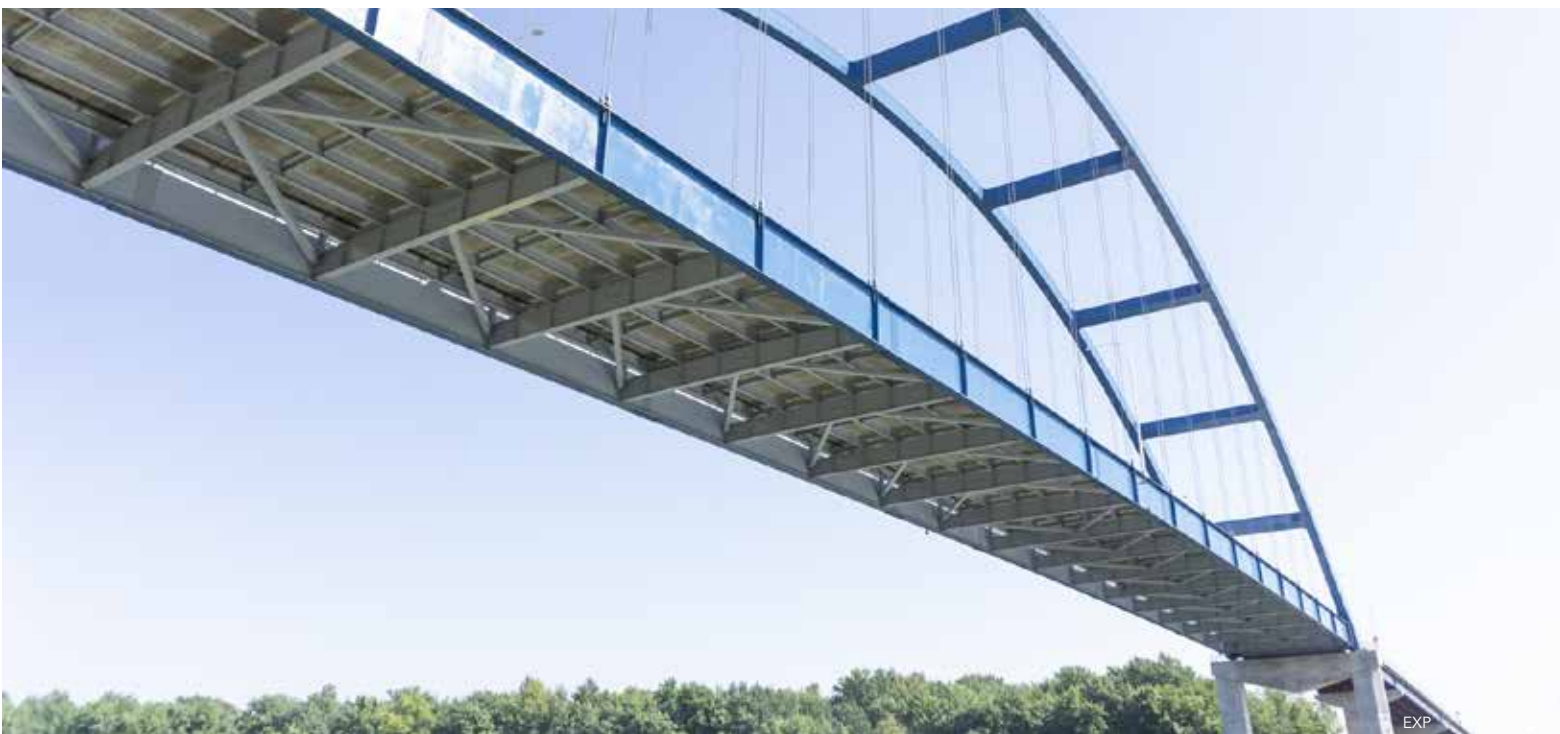
The new bridge carries two 12-ft lanes and two 10-ft shoulders and provides nearly 74 ft of vertical navigation clearance above normal pool. The bridge's design required complex analysis and used state-of-the-art programs to determine loads and perform design checks.
