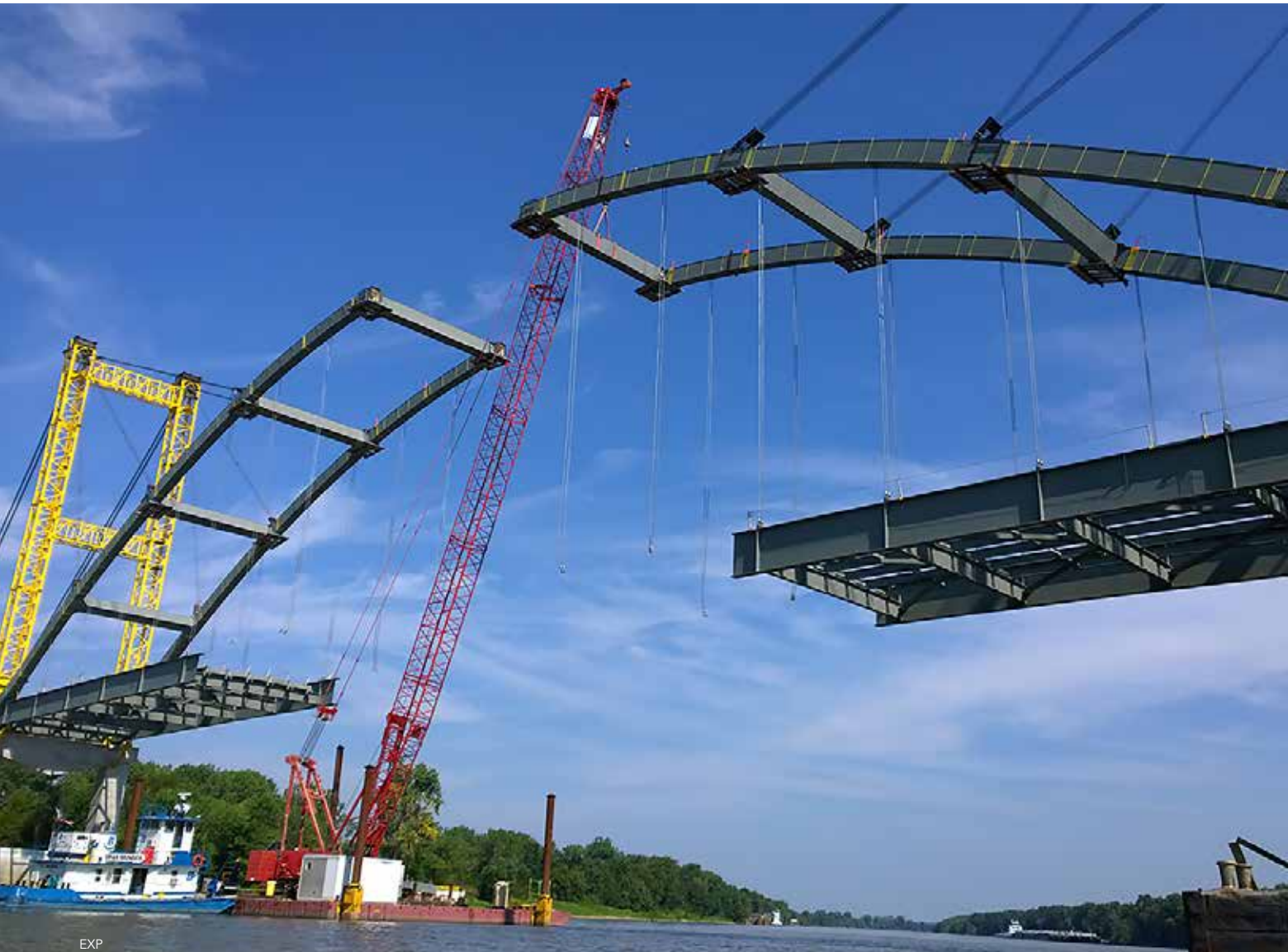
The main span of the bridge, coming together in the middle.
