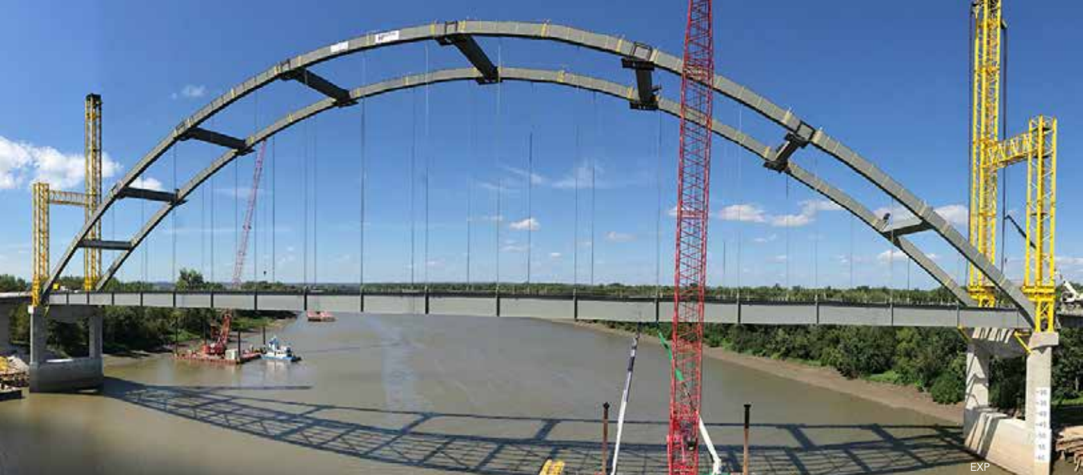
The new bridge carries two 12-ft lanes and two 10-ft shoulders and provides nearly 74 ft of vertical navigation clearance above normal pool. The bridge's design required complex analysis and used state-of-the-art programs to determine loads and perform design checks.
