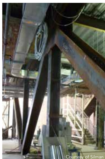
Multiple existing columns were removed at the first floor to create a new assembly space, and a story-deep truss was incorporated into a corridor wall on the floor above to transfer loads in the direction parallel to the long dimension of the new space.
