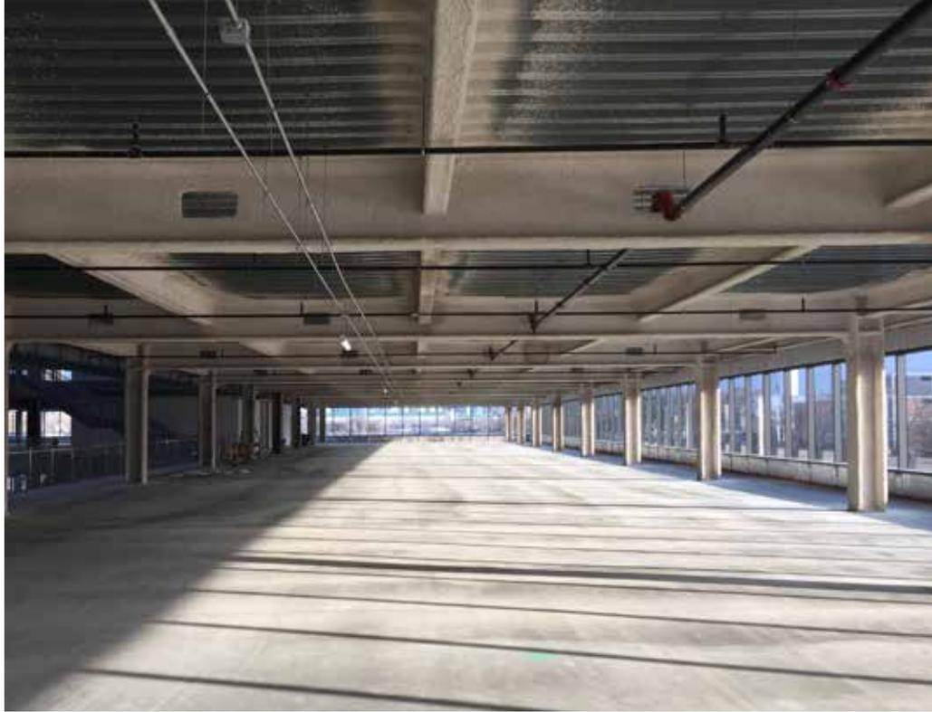
MEP services are integrated with the steel structure by providing shallower floor framing or web openings where required.
