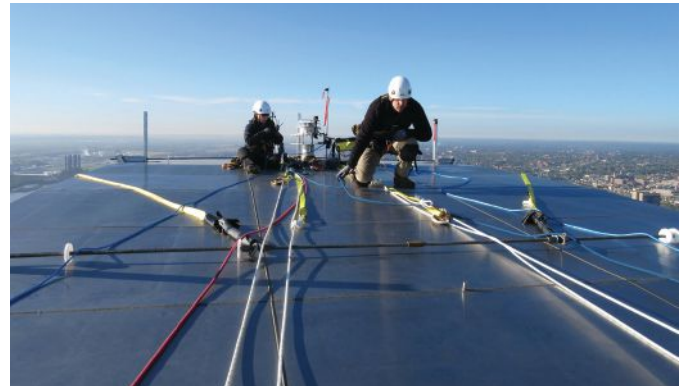
above: The primary anchor points for the rope system on top of the Arch. below: The rope system's secondary anchor point during installation.
