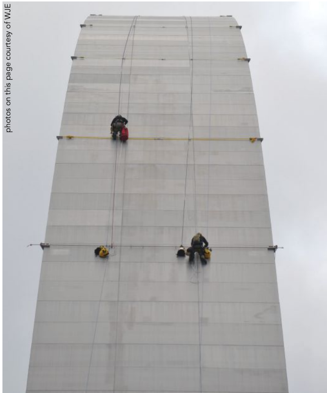
above: Using the industrial rope access system on the north leg. below: Access at the intrados.
