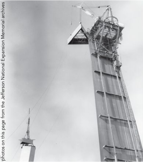
Placing a station of the Arch via creeper derrick crane.
