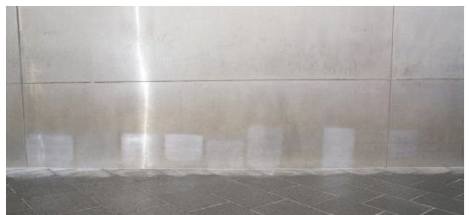
below: Cleaning-study test areas at the base of the Arch.
