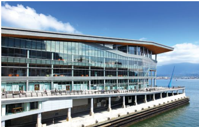
VANCOUVER CONVENTION CENTER EXPANSION PROJECT
