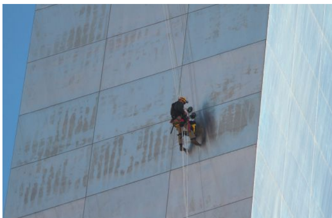
above: Using the industrial rope access system on the north leg. below: Access at the intrados.
