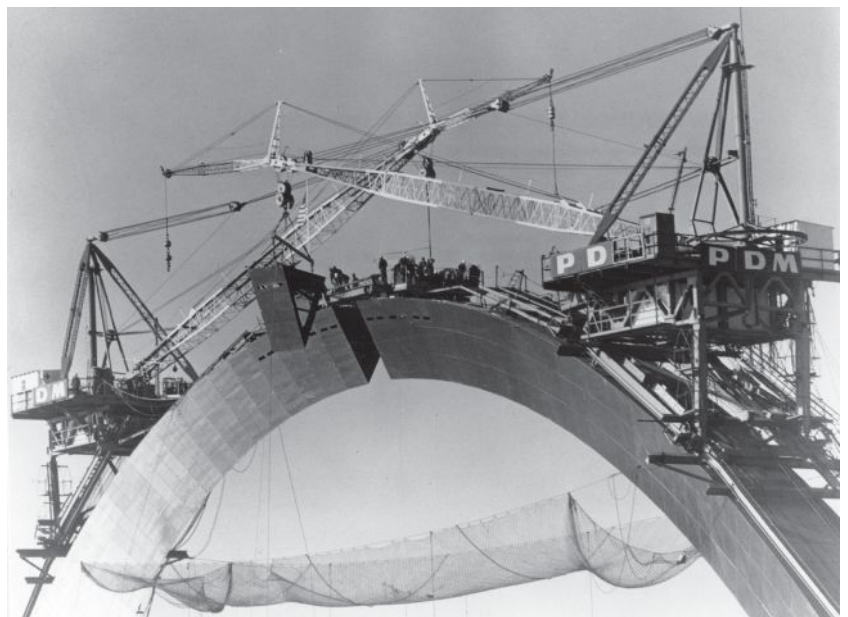
Installing a stabilizing strut to resist overturning and deflection of the cantilevered legs. Installing the final station of the Arch, at the top of the north leg, on October 28, 1965.
