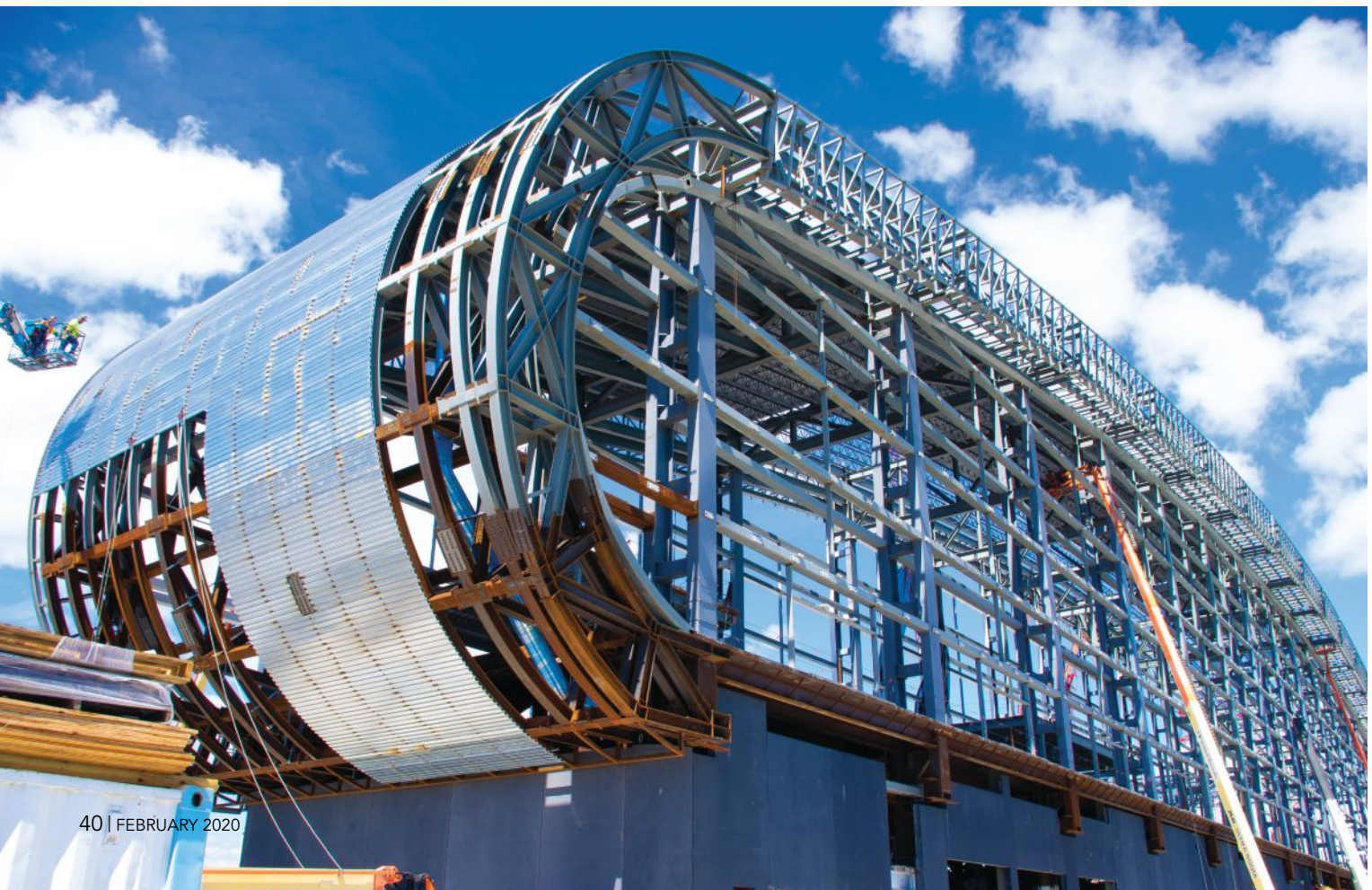
below: The curvaceous building is 128 ft tall at its peak and 800 ft long, comprising a total of 166,500 sq. ft. Norwegian required a taller terminal to accommodate boarding for its newer “super cruisers.”
