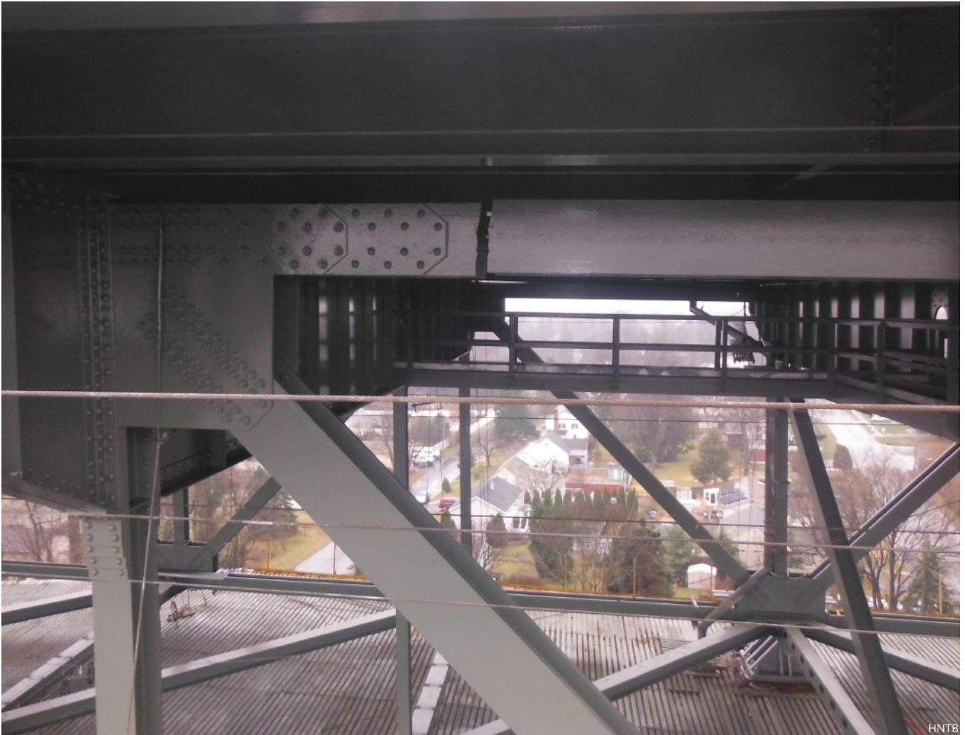
above and opposite page: A fracture of a fracture-critical-designated member on the Delaware River Turnpike Bridge, which continued to carry service loads until the fracture was discovered and repaired.
