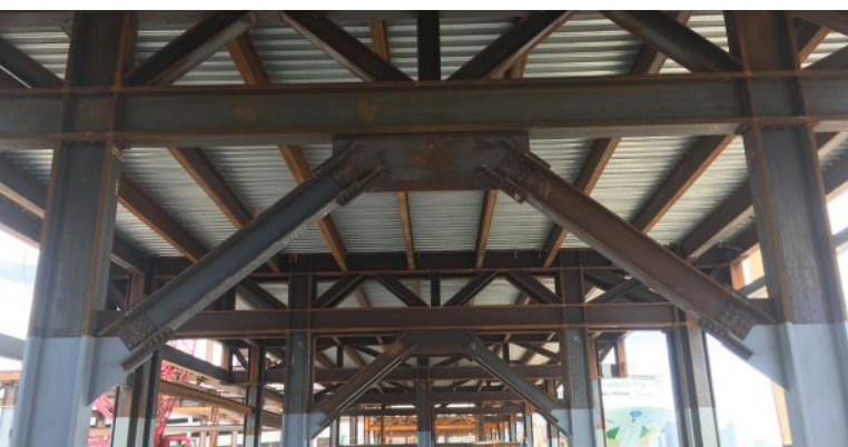
below: Support framing below one of the pearls.
